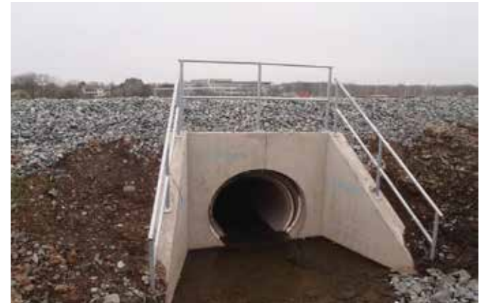
Outfall with Backflow Prevention (Flap Gate):
