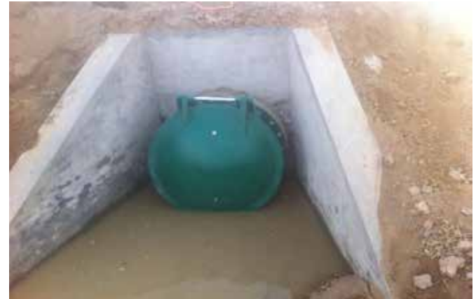
Outfall with Backflow Prevention (Flap Gate):
