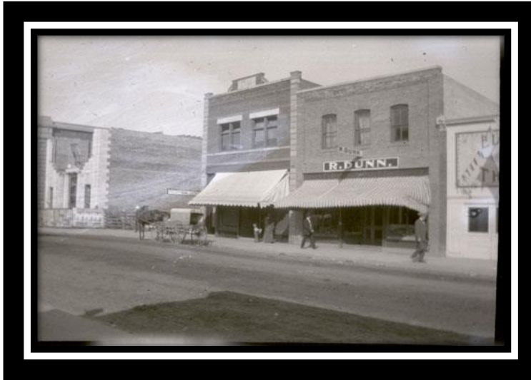
Merchants Bank under const. far left Bell Block to the left R. Dunn store to the right Electric Star Theatre far right 1909 0488-0006
