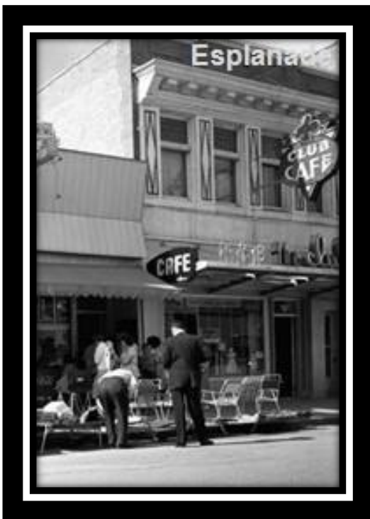
June, 1962: Original brick on front of building is exposed 942-A*
