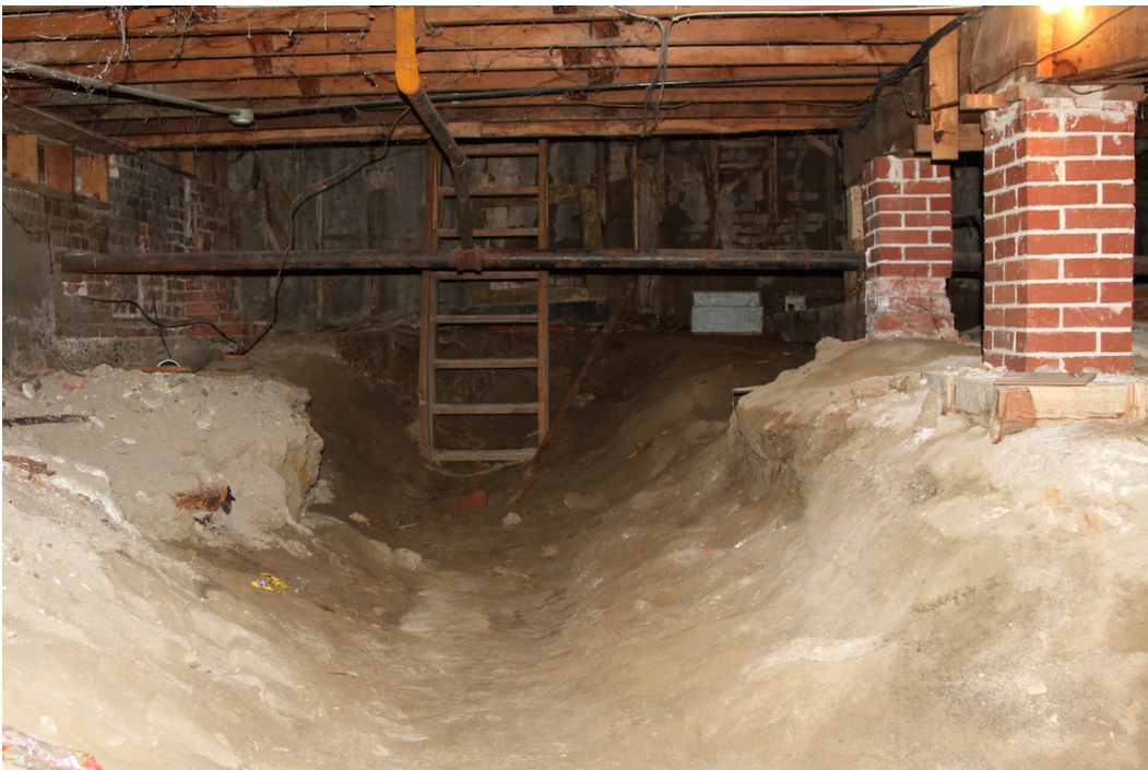
Basement showing masonry structural columns and wooden beams (Donald Luxton & Associates, 2014).
