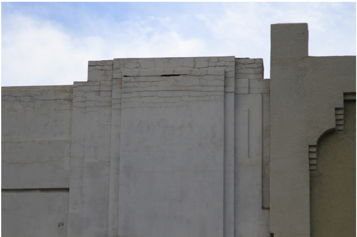
Monarch Theatre detail of vertical tower and damage to stucco cladding (Donald Luxton & Associates, 2014).
