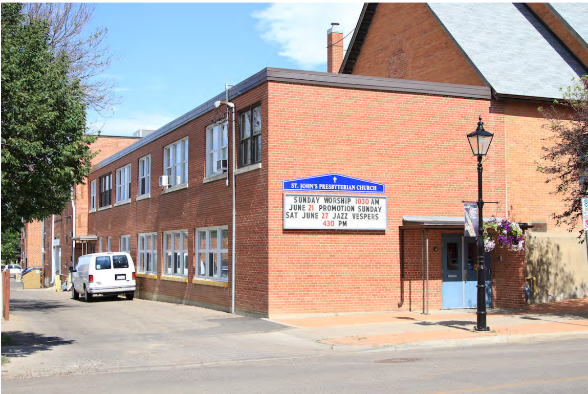
North façade of 1954 addition showing window replacement. Note infilled circular louvre in 1941 gabled addition, June 2015 (DLA)
