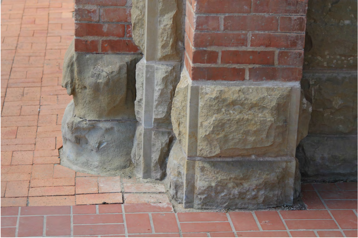
Sandstone foundation showing salt damage and replaced portion, June 2015 (DLA)
