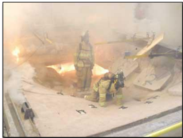
Figure 3: Floor Joist Collapse (National Research Council of Canada)
