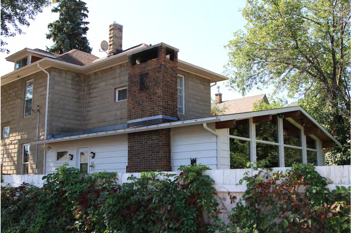
East and north façades showing 1972 addition, 2014 (DLA)
