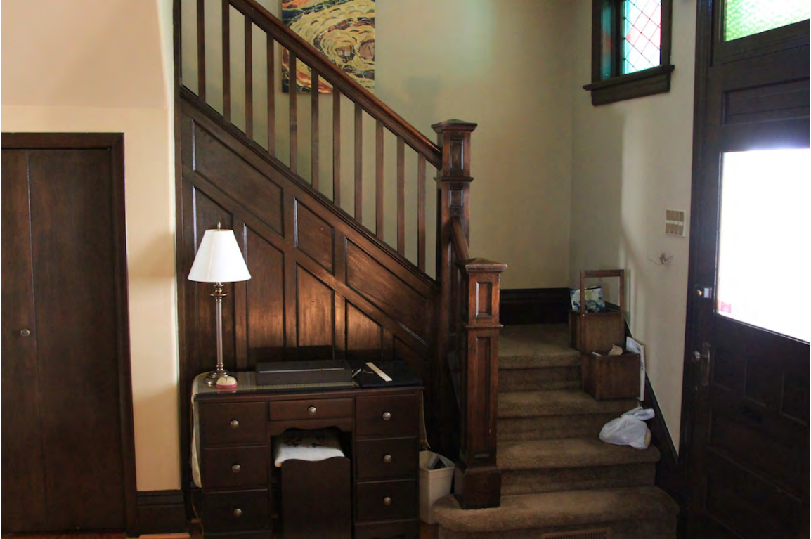
Staircase to second floor with wooden newel post and square wooden spindles, 2014 (DLA)
