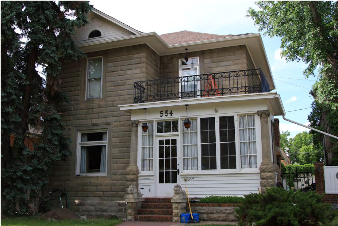
Front façade showing later enclosed front porch, and replaced balcony balustrade and entry stairs, 2014 (DLA)
