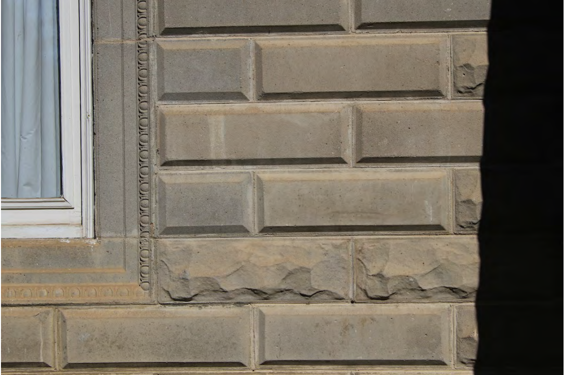
Moulded window casing with egg and dart, smooth moulded concrete block with rough finished moulded concrete block at sill height, 2014 (DLA)
