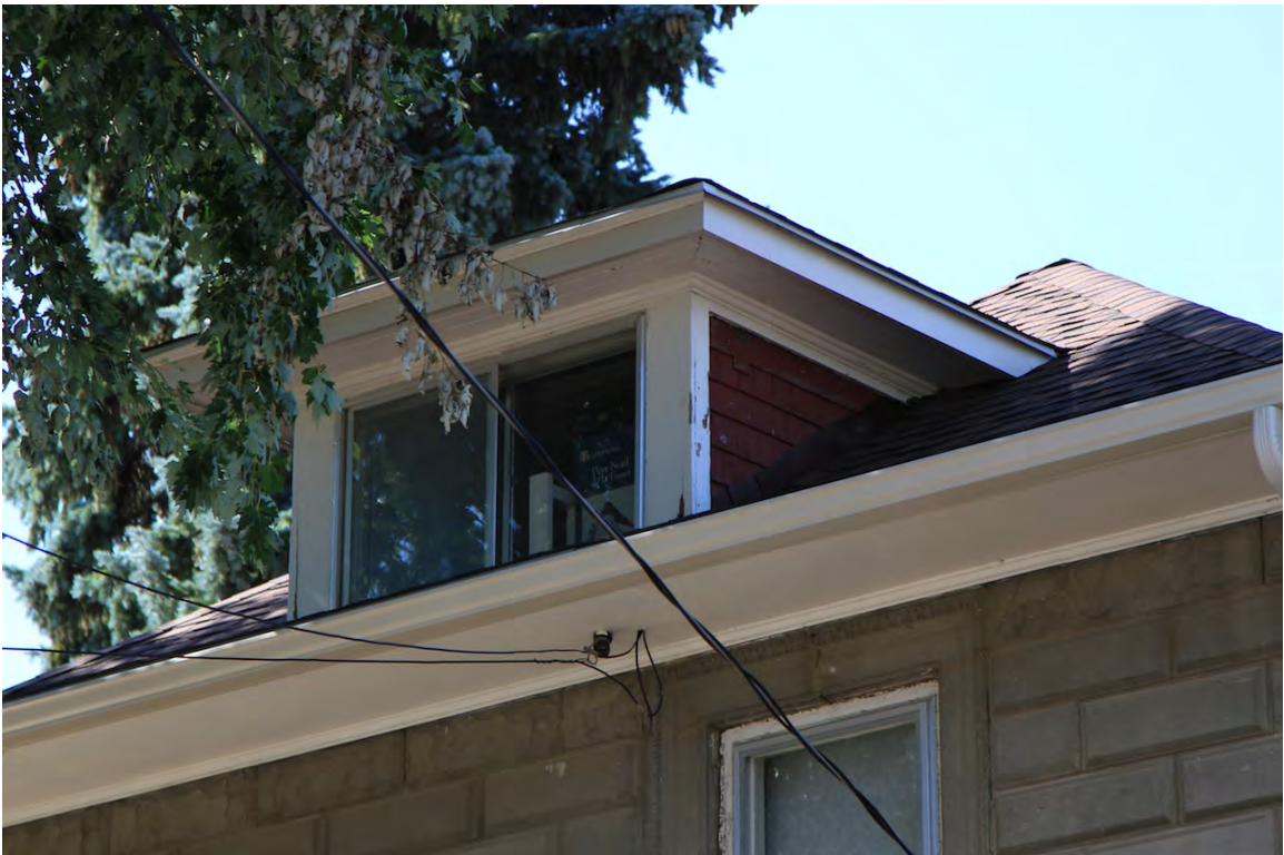
Hipped roof dormer with shingle cheeks and tongue and groove soffits, 2014 (DLA)
