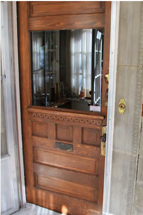
Eastlake-style wooden front door with mould concrete casing with egg and dart detail, 2014 (DLA)
