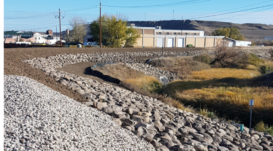
Flood mitigation berm and stormwater outfall near Industrial Avenue SE.
