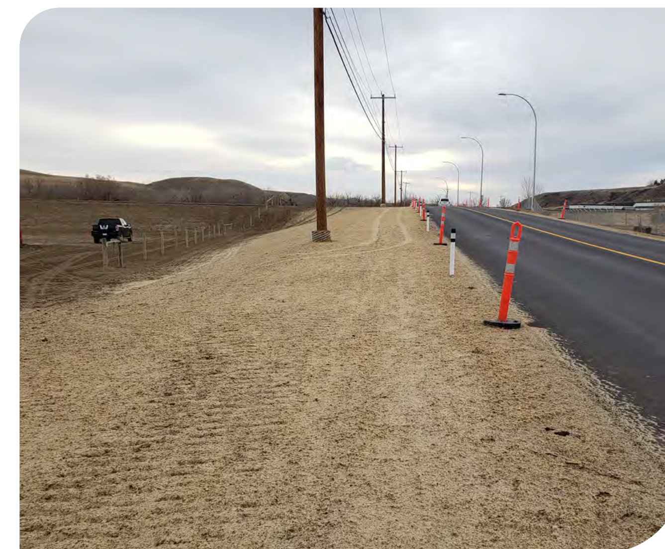
Industrial Ave berm looking east
