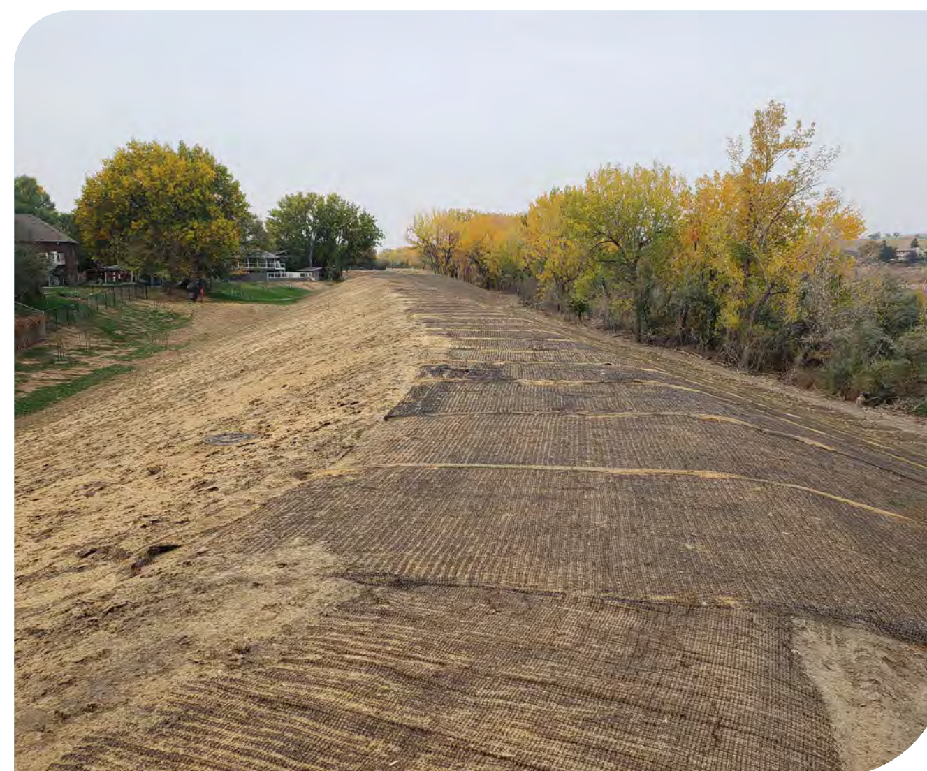
Phase 2 of the Harlow berm looking west
