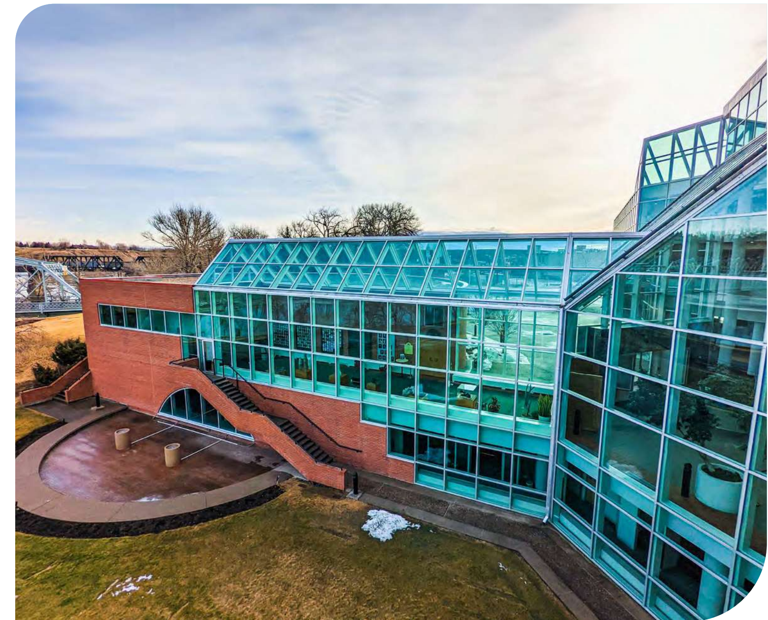
View of the Legislative Hallway with atrium on the right
