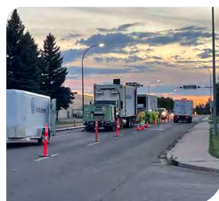
SOUTHVIEW DRIVE SEWER LINING PROJECT
