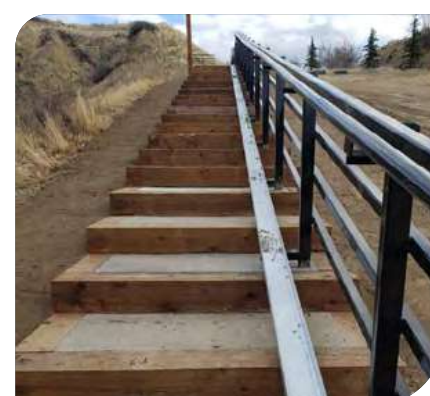
STAIRS IN KIN COULEE PARK
