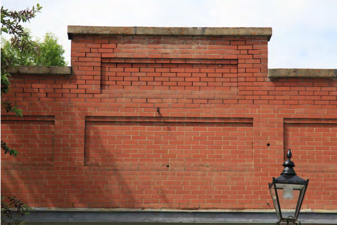
Stepped parapet showing missing mortar, 2014 (DLA)
