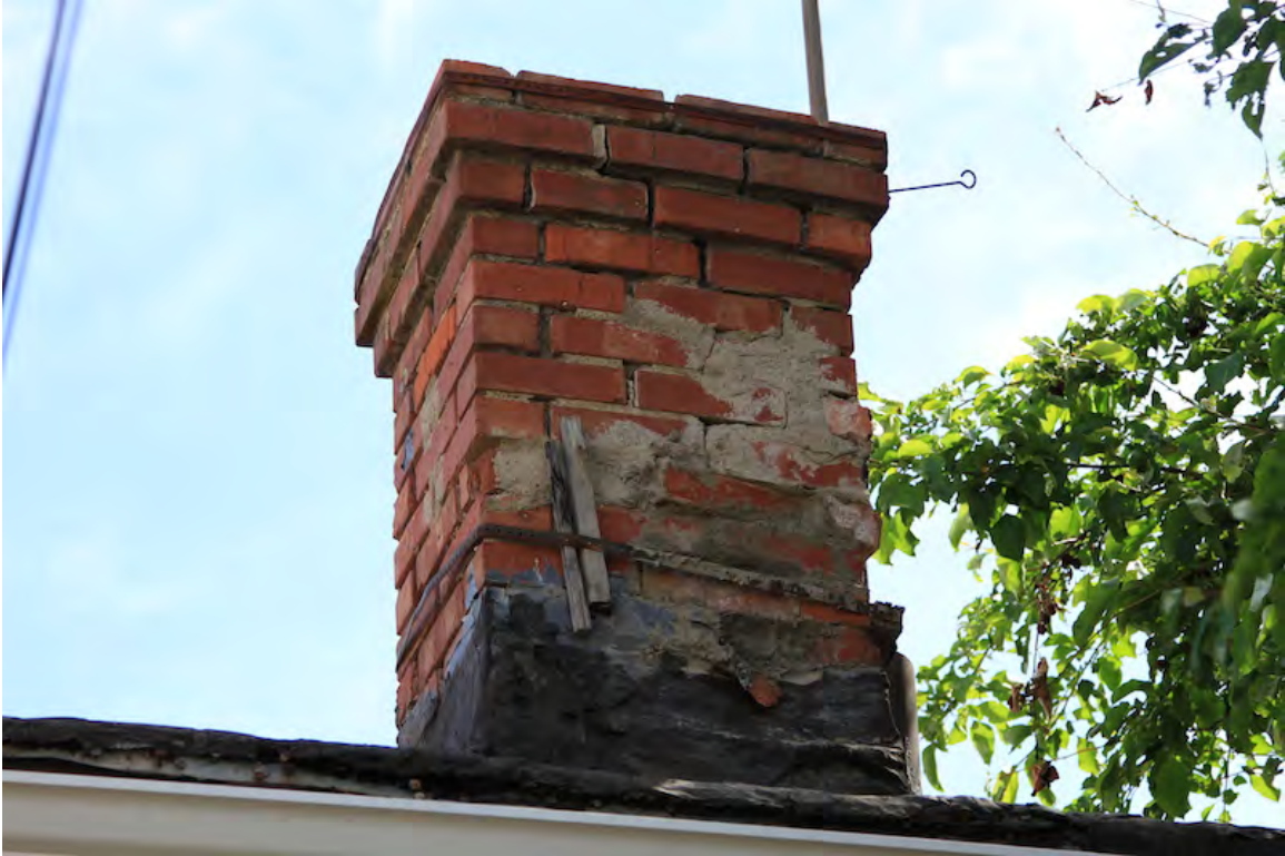
Rear chimney with missing mortar, 2014 (DLA)
