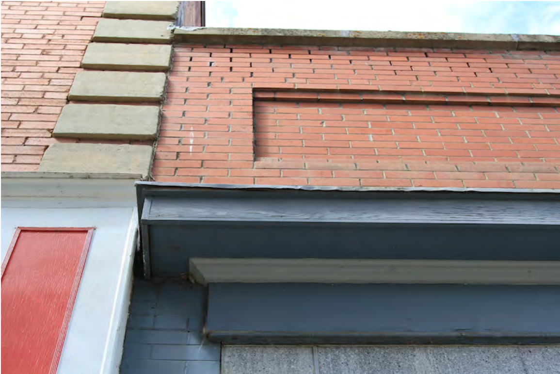
Storefront cornice with removed frieze and recessed panels above, 2014 (DLA)
