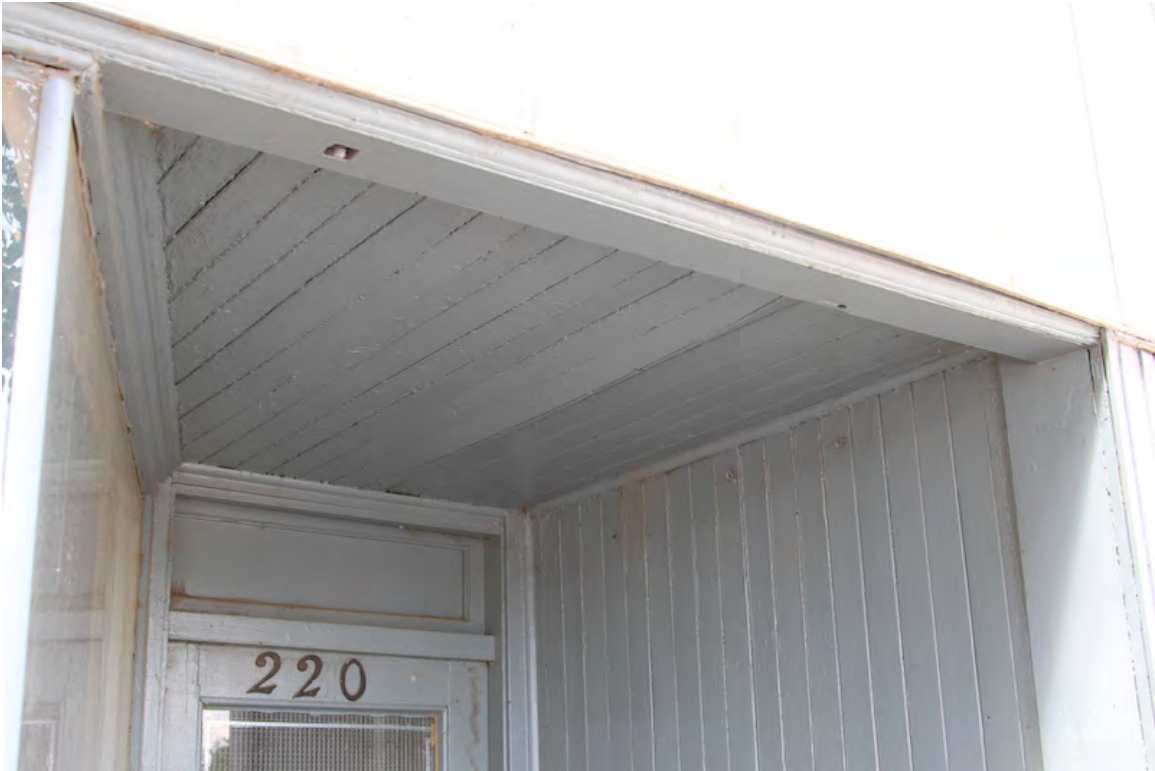
Original wooden soffit in storefront entryway, Suite 220, 2014 (DLA)
