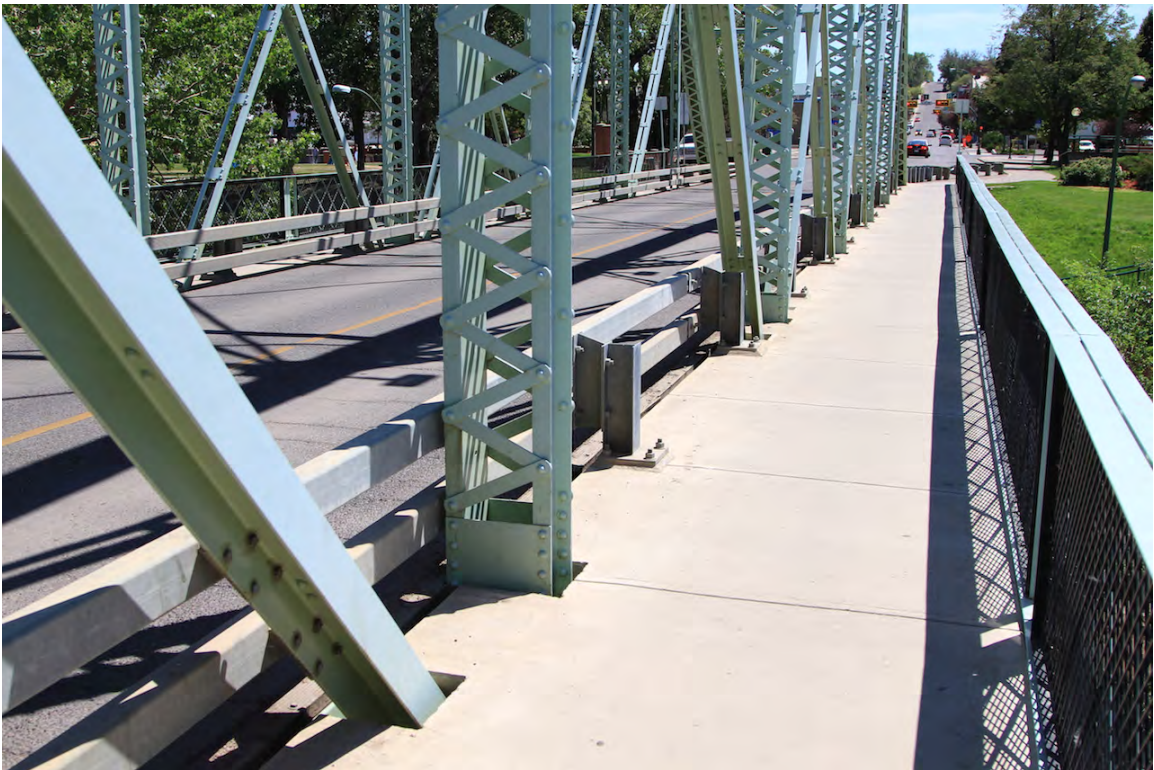
Pedestrian sidewalk adjacent to traffic lanes, June 2015 (DLA)
