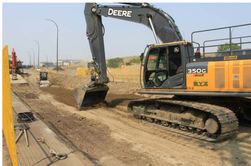
Construction of the first phase (2018) of a major sanitary sewer trunk line replacement project which will eventually extend east to west across all of Riverside.
