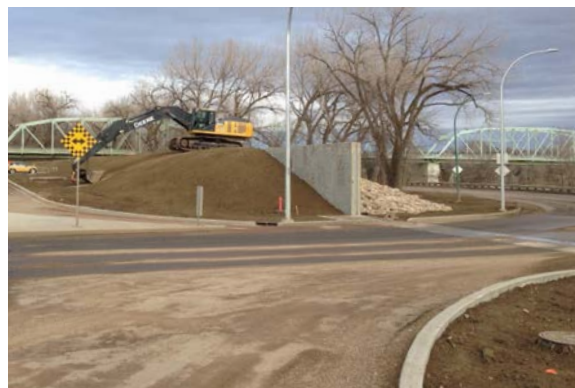
Parkview Drive NE, during 2017 construction of flood mitigation berm.
