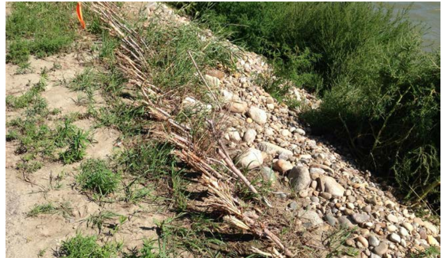
Riverbank erosion control using live stakes (recreational trail near Garden Place NW).
