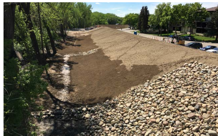
Riverside flood mitigation berm, shortly after construction in 2017.
