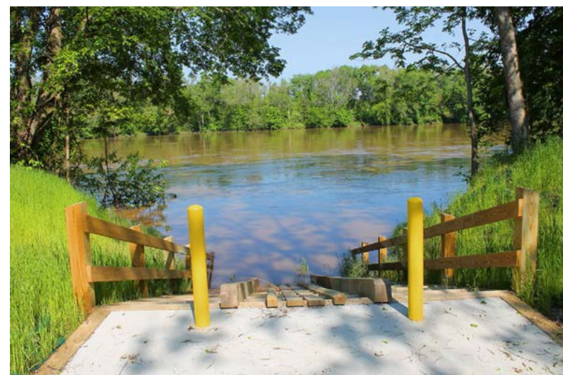
Example of boat launch for kayaks and canoes. Bollards prevent launching of motorized watercraft.
