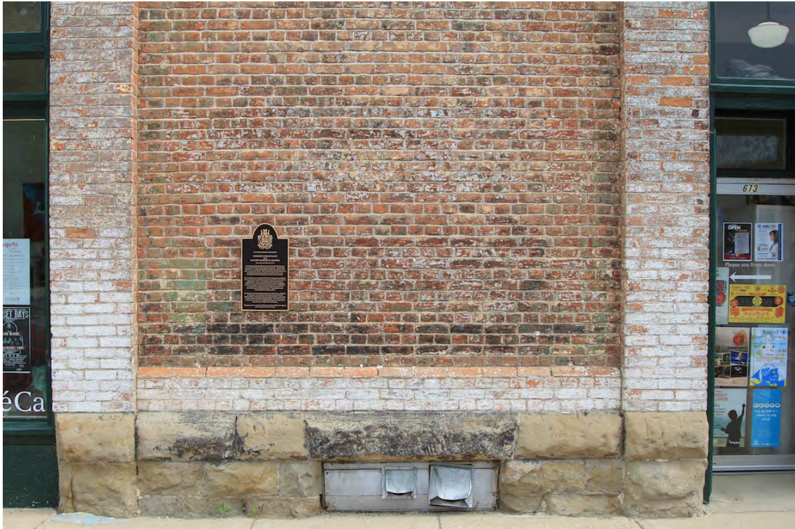
Brick façade with MHR plaque and showing both sandstone deterioration and results of paint removal from brick, June 2015 (DLA)
