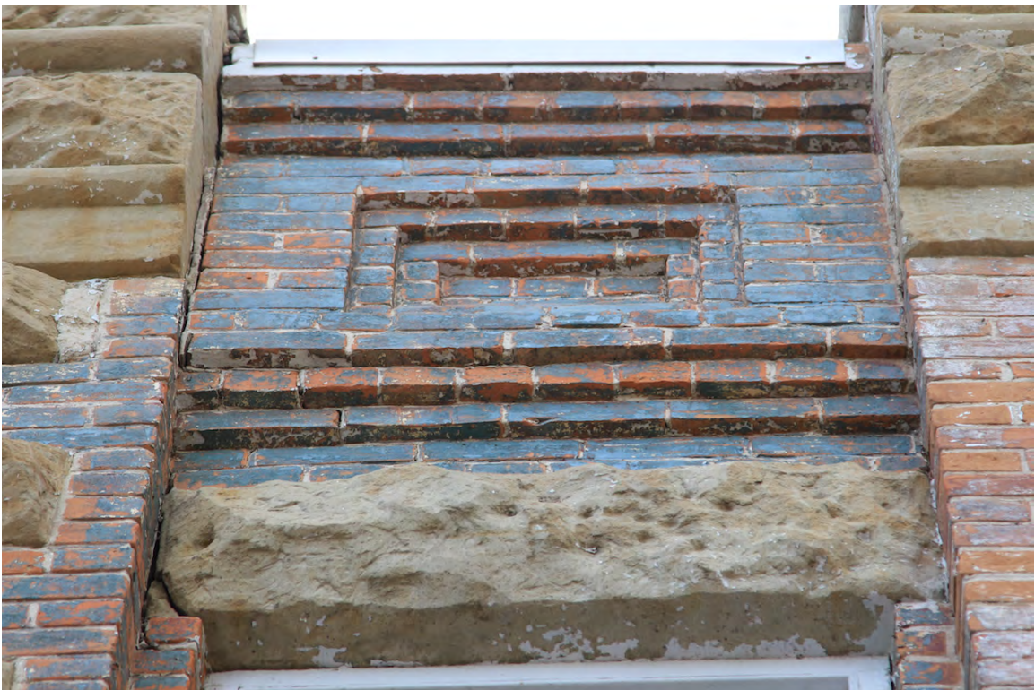
Decorative corbelled brick panel below corbelled brick parapet with metal cap flashing, June 2015 (DLA)
