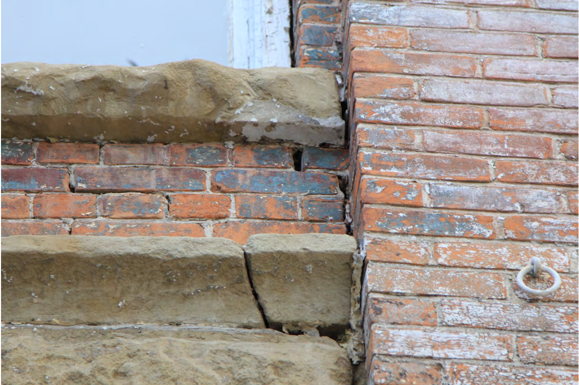
Cracked sandstone lintel, mortar loss, settlement issues at work, June 2015 (DLA)
