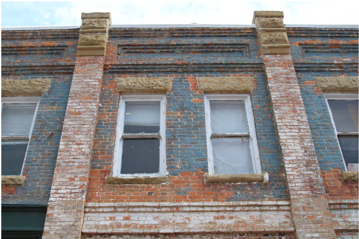
Single assembly, 1-over-1 single-hung wooden-sash windows on second storey, June 2015 (DLA)
