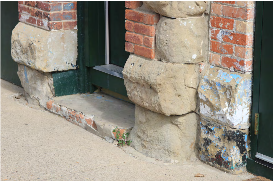
Deteriorated sandstone water table with mortar loss, and damaged parging on brick stoop, June 2015 (DLA)
