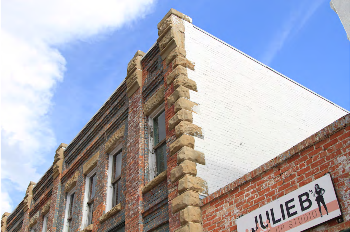
Sandstone quoining, sills, lintels, and pilaster cap of commercial block and painted west wall, June 2015 (DLA)
