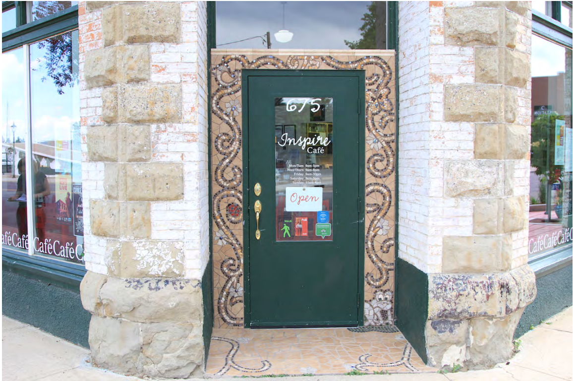
Chamfered entry with deteriorated sandstone watertable, replaced transom, covered sidelights, and replaced door, June 2015 (DLA).
