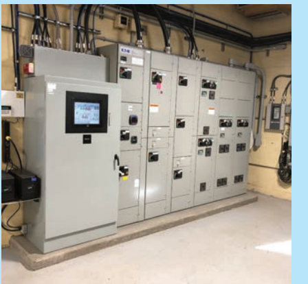
Final Effluent Pump House Motor Control Centre
