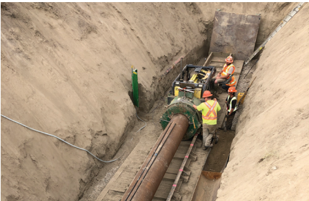
Auger bore machine at work
