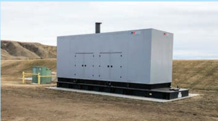
800 kW standby generator
