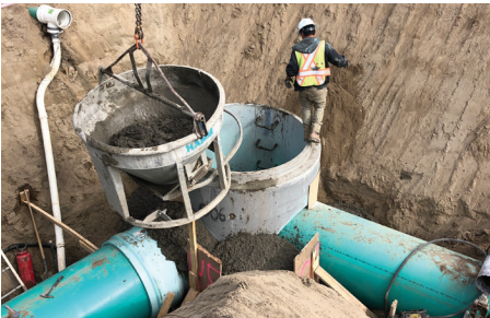
Manhole installation on large diameter (1050 mm) sanitary sewer pipe
