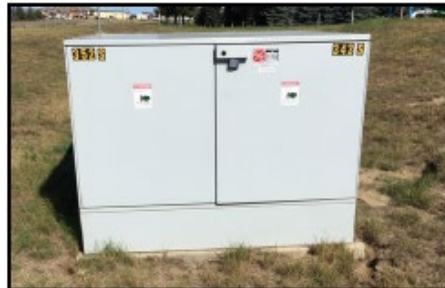
Padmount Switchgear
