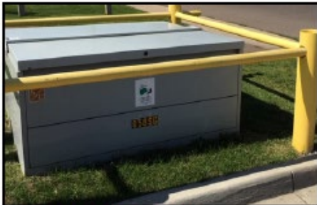
Padmount Switchgear
