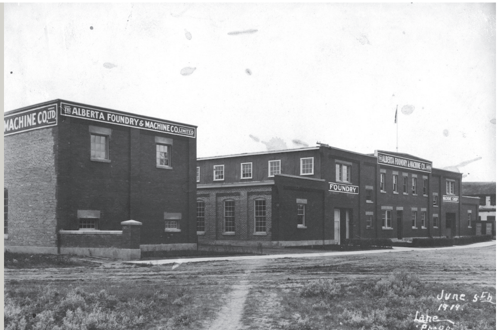
1919 photo of the 1916 Alberta Foundry & Machine Shop which encapsulated the original 1911-1914 iron and wood frame structures
