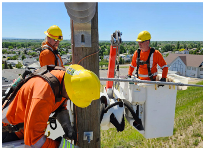
Utility line workers perform overhead line work on a wooden utility pole. The City of Medicine Hat is the electricity source, transmitter, distributor, and the retailer for the community.
