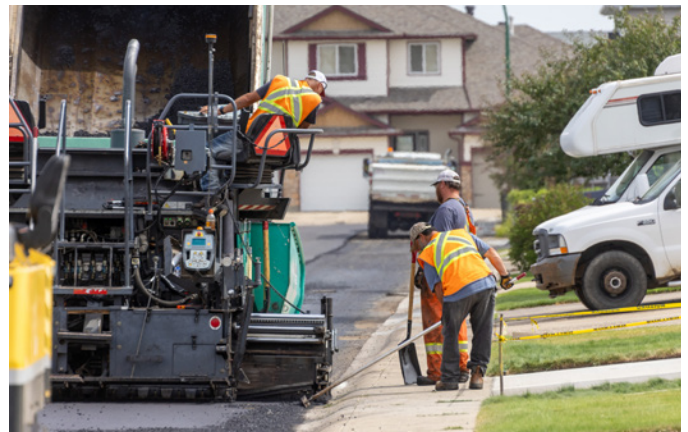
A road resurfacing crew laying fresh asphalt on a residential street.
