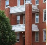
• Masonry construction including: concrete foundation; stretcher pattern pressed red brick exterior with red mortar; internal brick chimney
