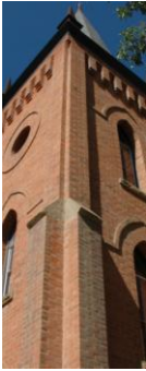
Photograph showing the engaged buttresses
