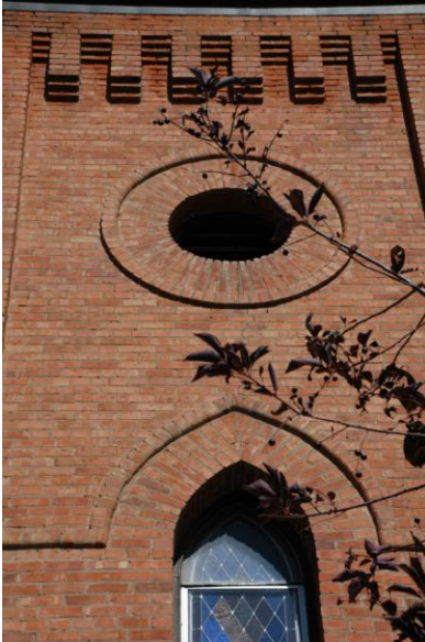
Photograph showing the small round brick vent details
