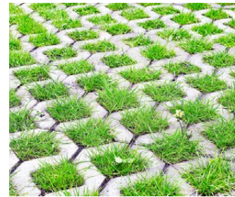
Semi-permeable concrete allows more water infiltration.
