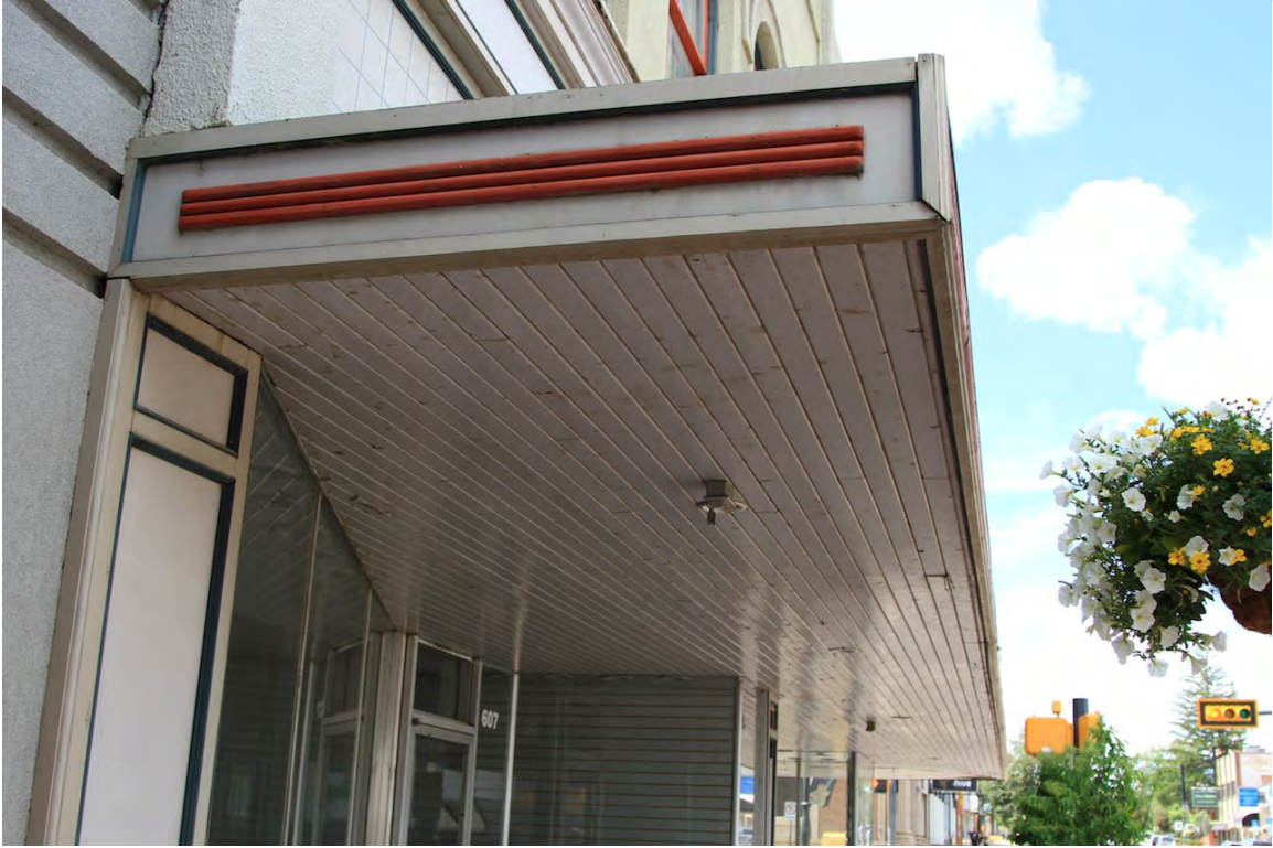
1951 canopy with tongue and groove wooden soffit, 2014 (DLA)
