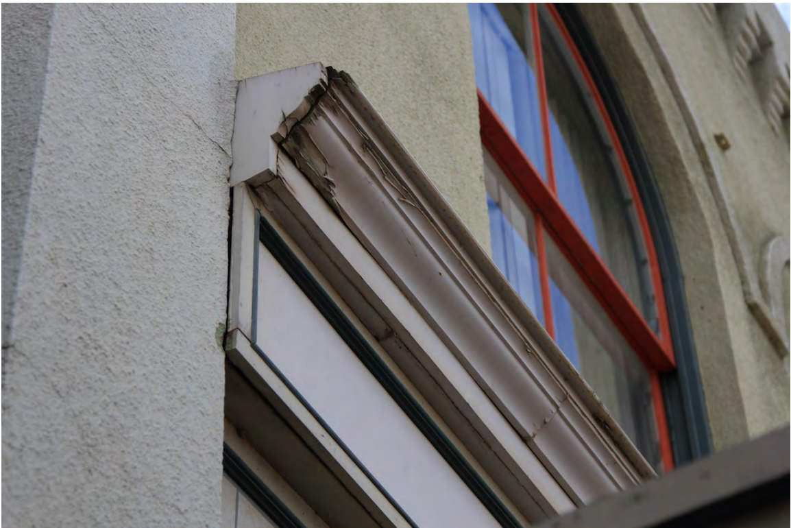
Wooden storefront cornice exhibiting paint loss and water damage, 2014 (DLA)
