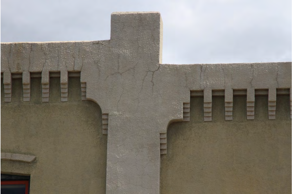
Cracks in parapet stucco, 2014 (DLA)
