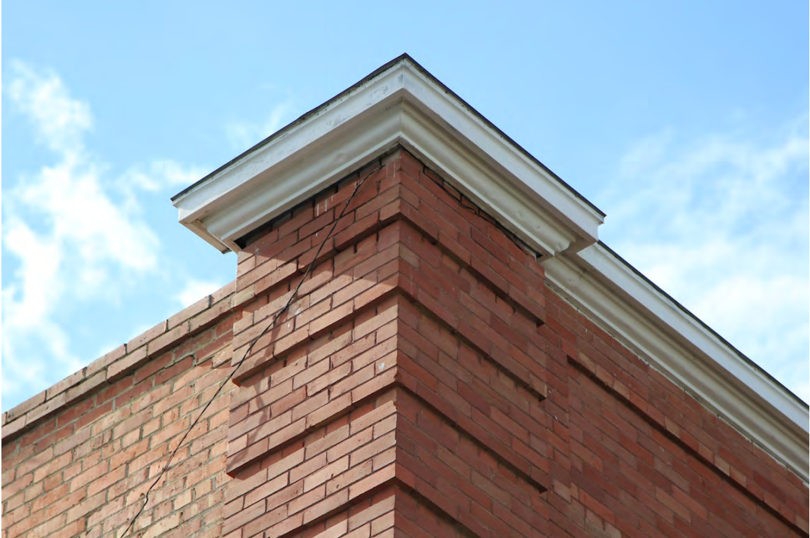
Corbelled wooden parapet cap on front façade, June 2014 (DLA)
