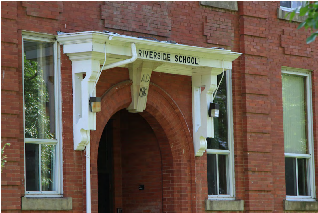
Decorative wooden entry cornice with brackets over recessed central entry with flat brick arch with voussoir, June 2014 (DLA)
