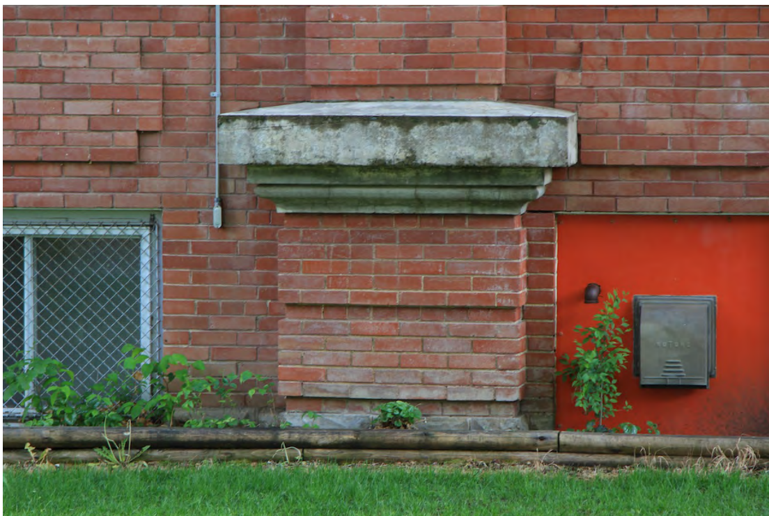
Molded concrete base at banded brick pilaster, June 2014 (DLA)
