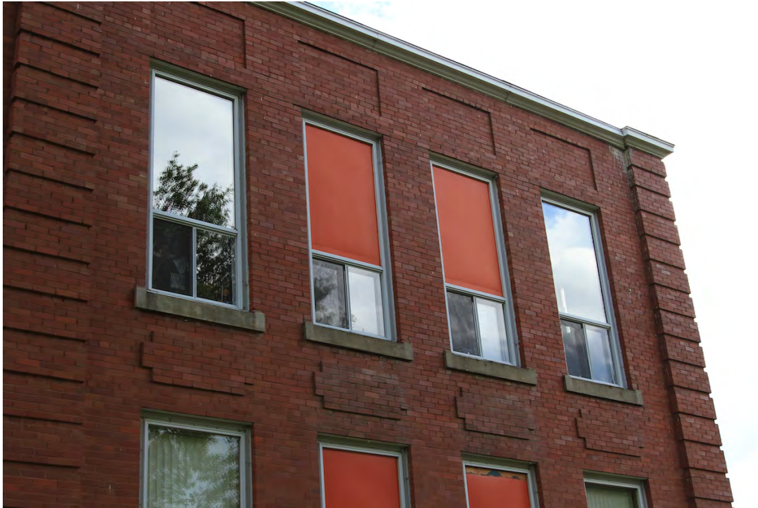
Regular fenestration with concrete sills, with decorative brick relief above and below, June 2014 (DLA)
