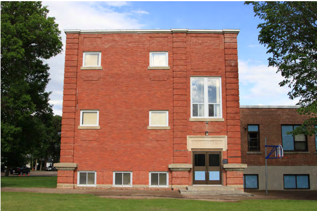
Side façade showing banded brick pilasters on mold concrete bases with single and double assembly window openings, June 2014 (DLA)
