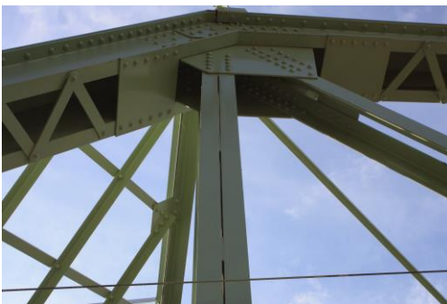
Photographs showing the riveted steel construction on Finlay Bridge
