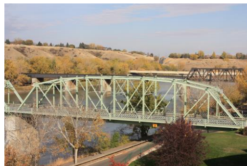
Photographs showing a span of the curved chord Pratt trusses
