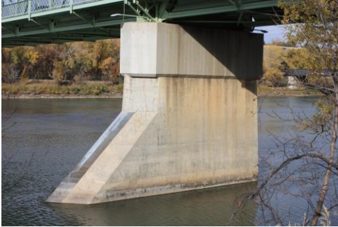
Photographs showing the cast-in-place concrete piers and abutments
