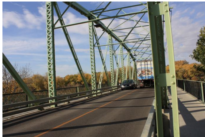
Photographs showing the continuous use, riveted steel construction, curved chord Pratt trusses
