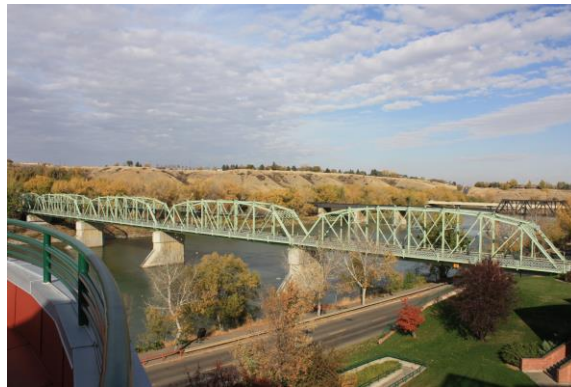
Photograph showing five spans of curve chord Pratt trusses
