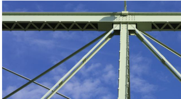
Photographs showing the riveted steel construction on Finlay Bridge
