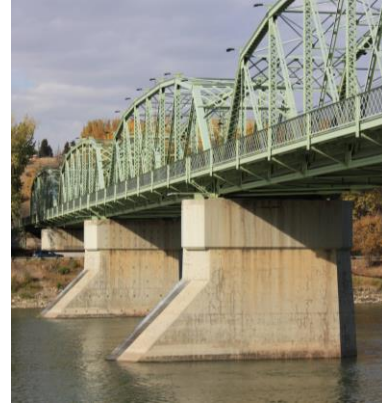
Photographs showing the cast-in-place concrete piers and abutments
