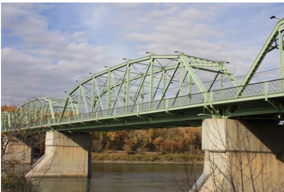
Photographs showing a span of the curved chord Pratt trusses
