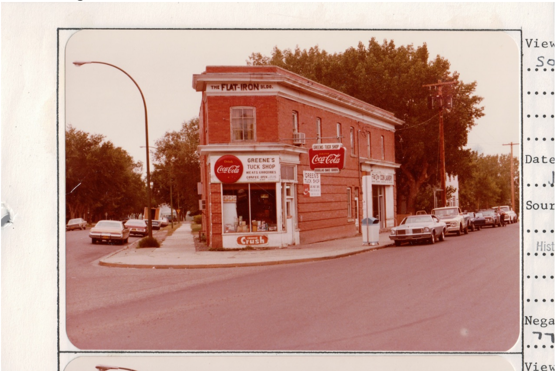
Greene's Tuck Shop (Flat Iron Building), 1977 (Historic Sites Alberta)
