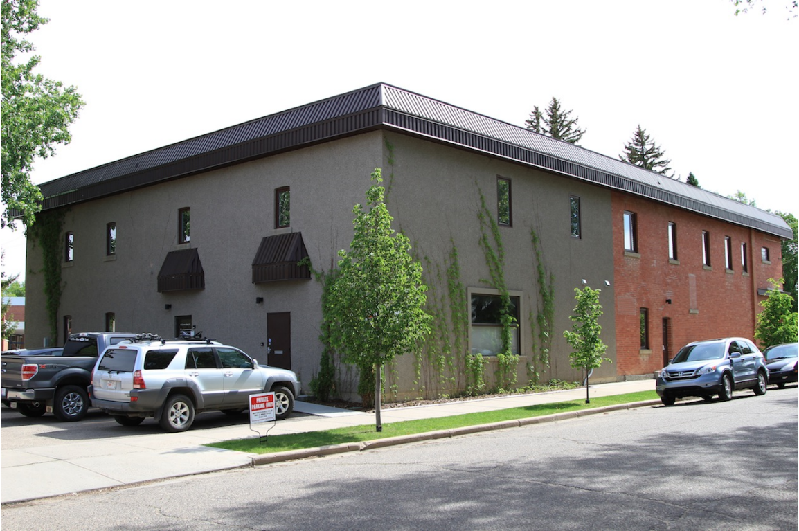
Rear of two-storey addition and connection to original building on north façade, 2014 (Donald Luxton & Associates)
