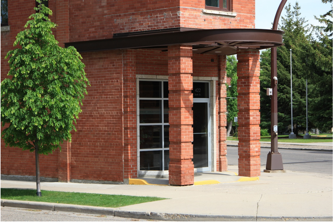
Reconfigured former storefront with original and additional brick column and new recessed entry, 2014 (Donald Luxton & Associates)
