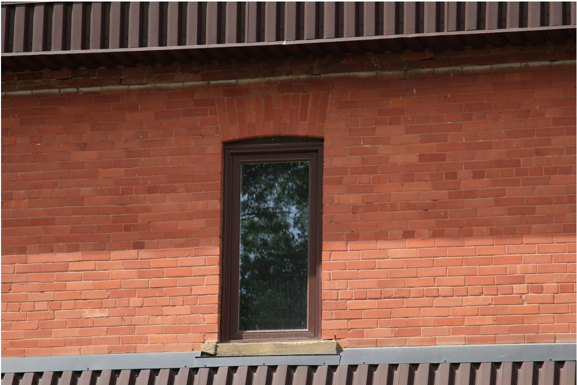
Replaced window, with original window opening maintained, 2014 (Donald Luxton & Associates)
