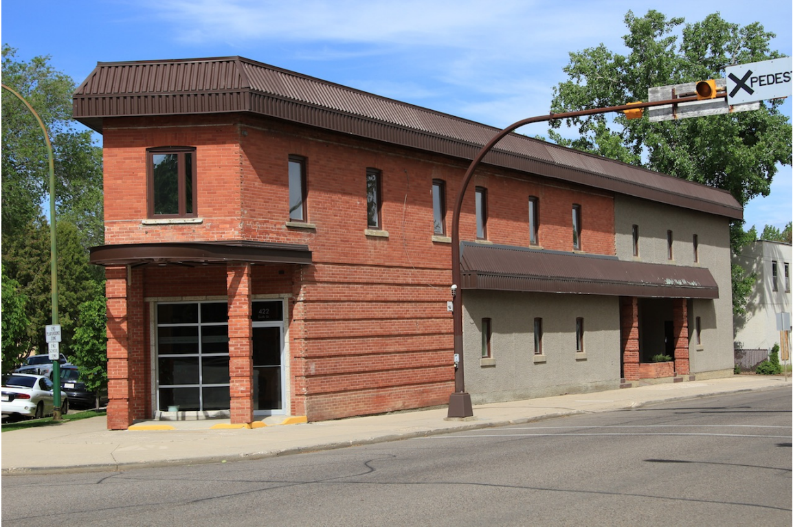
South façade showing two-storey addition at rear and infilled and re-clad second storefront location, 2014 (Donald Luxton & Associates)
