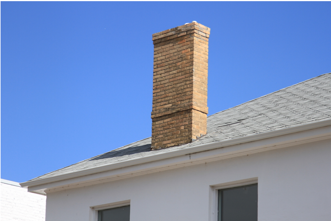
Brick chimney with corbelled cap, June 2015 (DLA)
