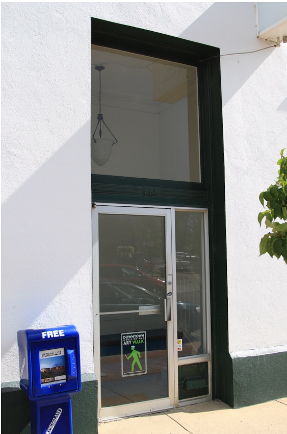
Original entry with intact wooden-sash single light transom, June 2015 (DLA)
