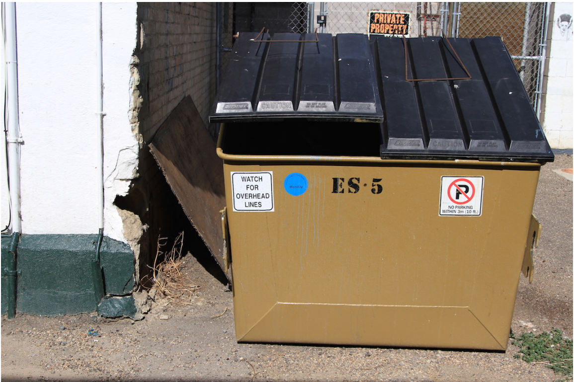
Damage to sandstone quoining at southwest corner of building, June 2015 (DLA)
