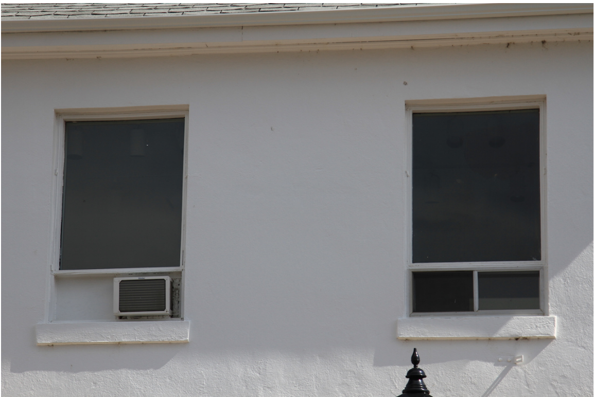
Rectangular window openings with parged stone sills on second storey, windows replaced, June 2015 (DLA)
