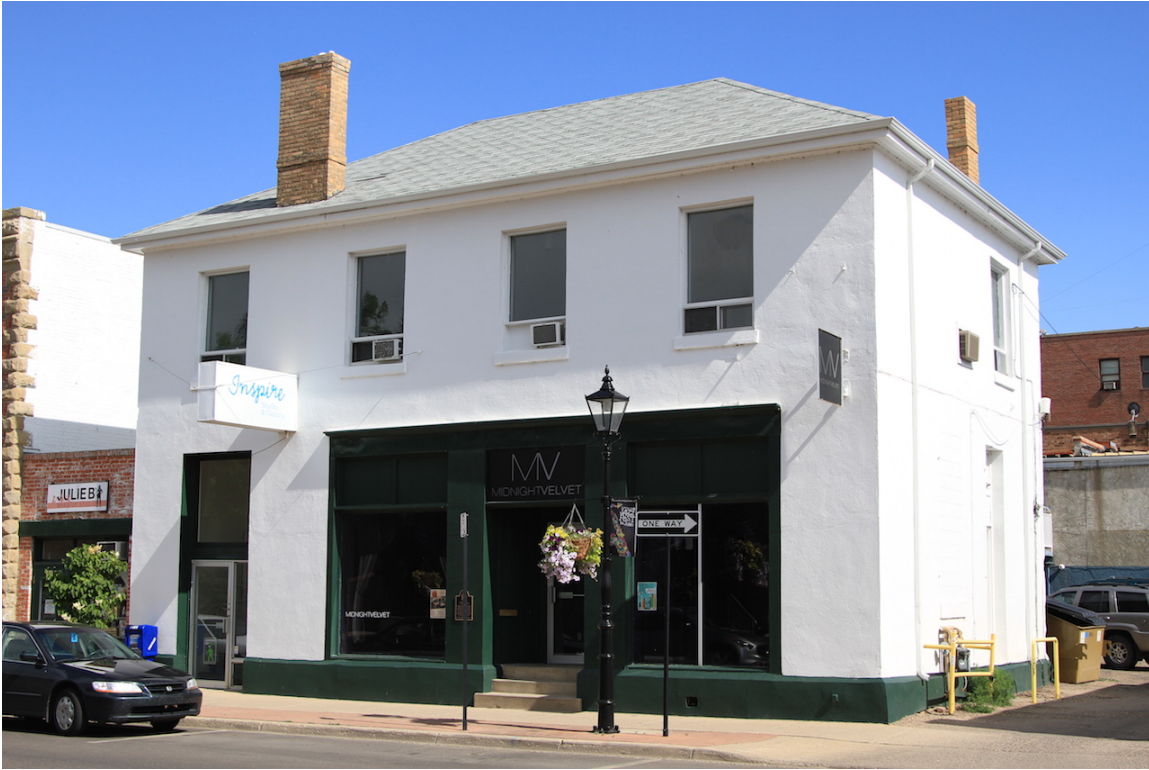
Stucco clad north and east façades and later added storefront on north façade, June 2015 (DLA)
