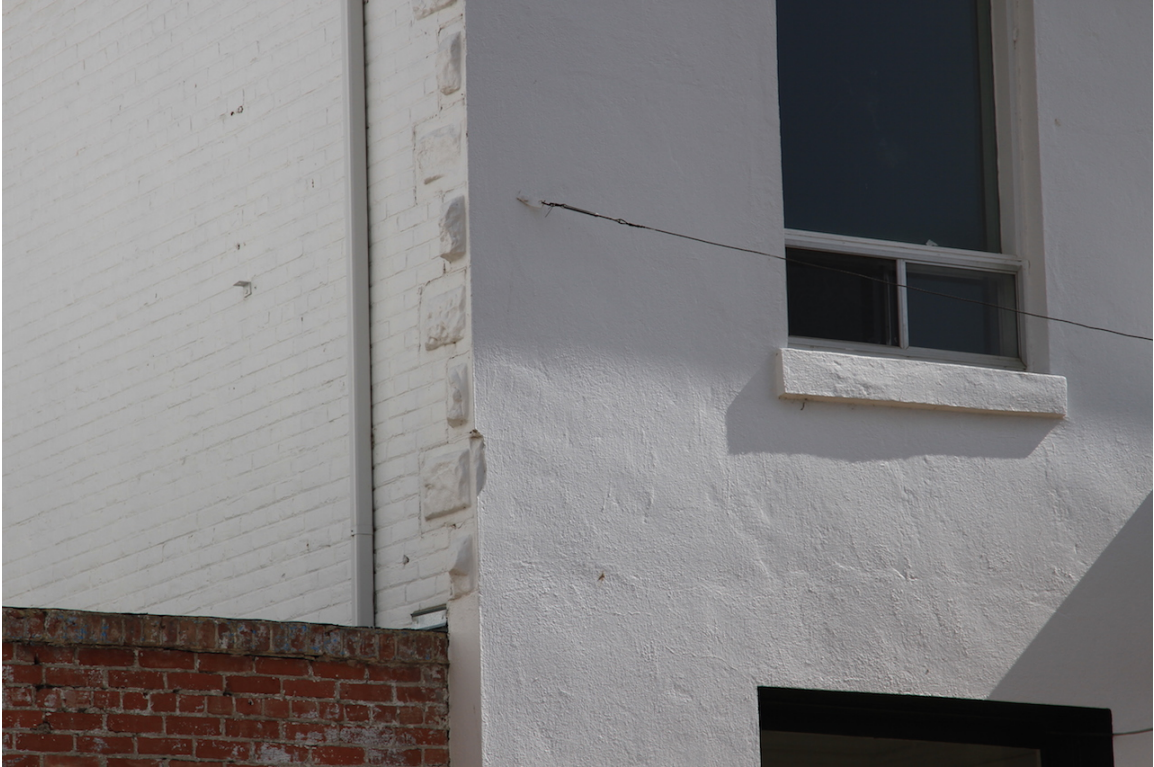
Original brick exterior with sandstone quoining and later applied stucco, June 2015 (DLA)
