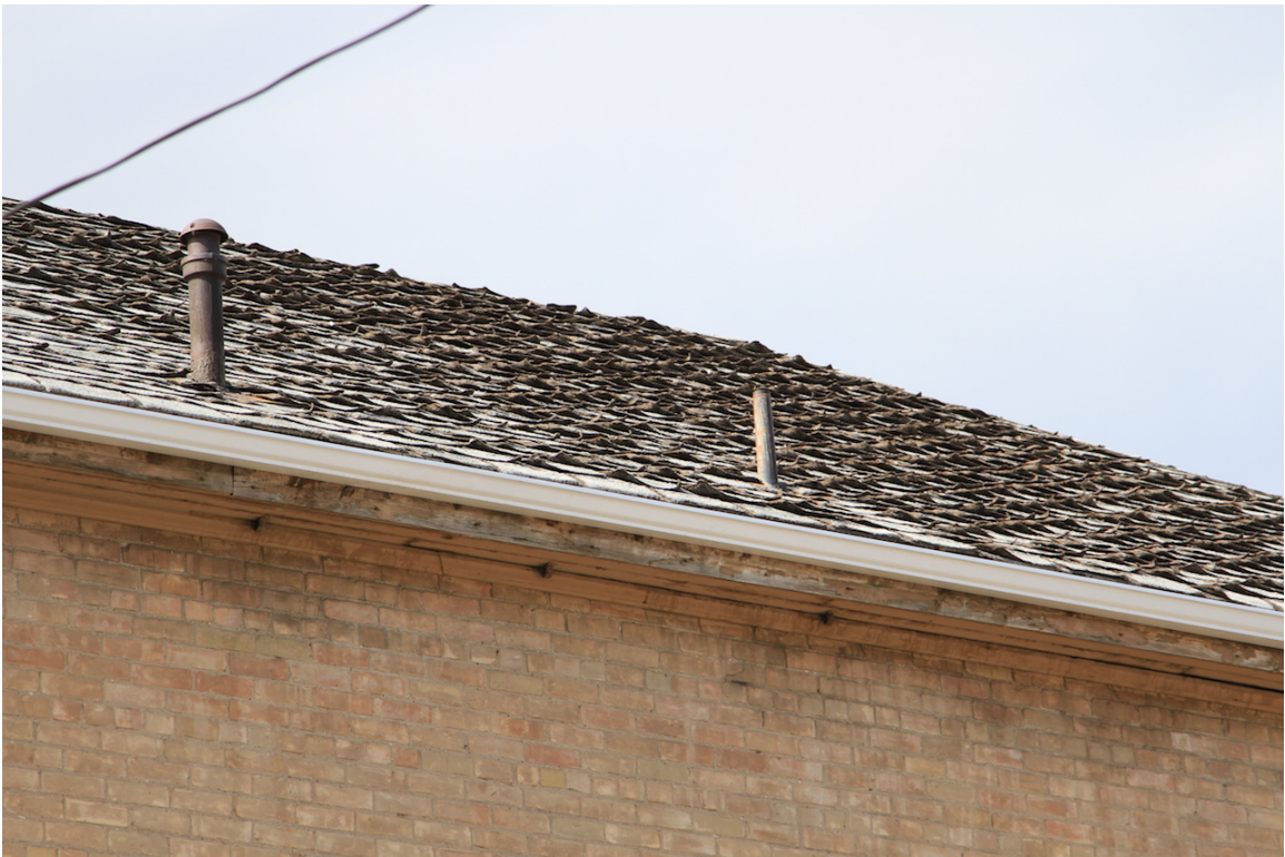
Deteriorated roof shingles on rear of roof, June 2015 (DLA)
