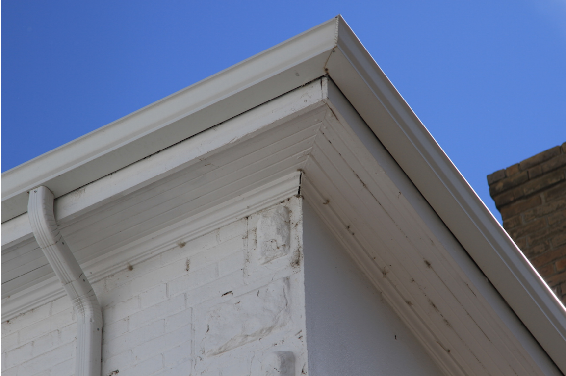
Wooden tongue and groove soffit with cornice board, June 2015 (DLA)
