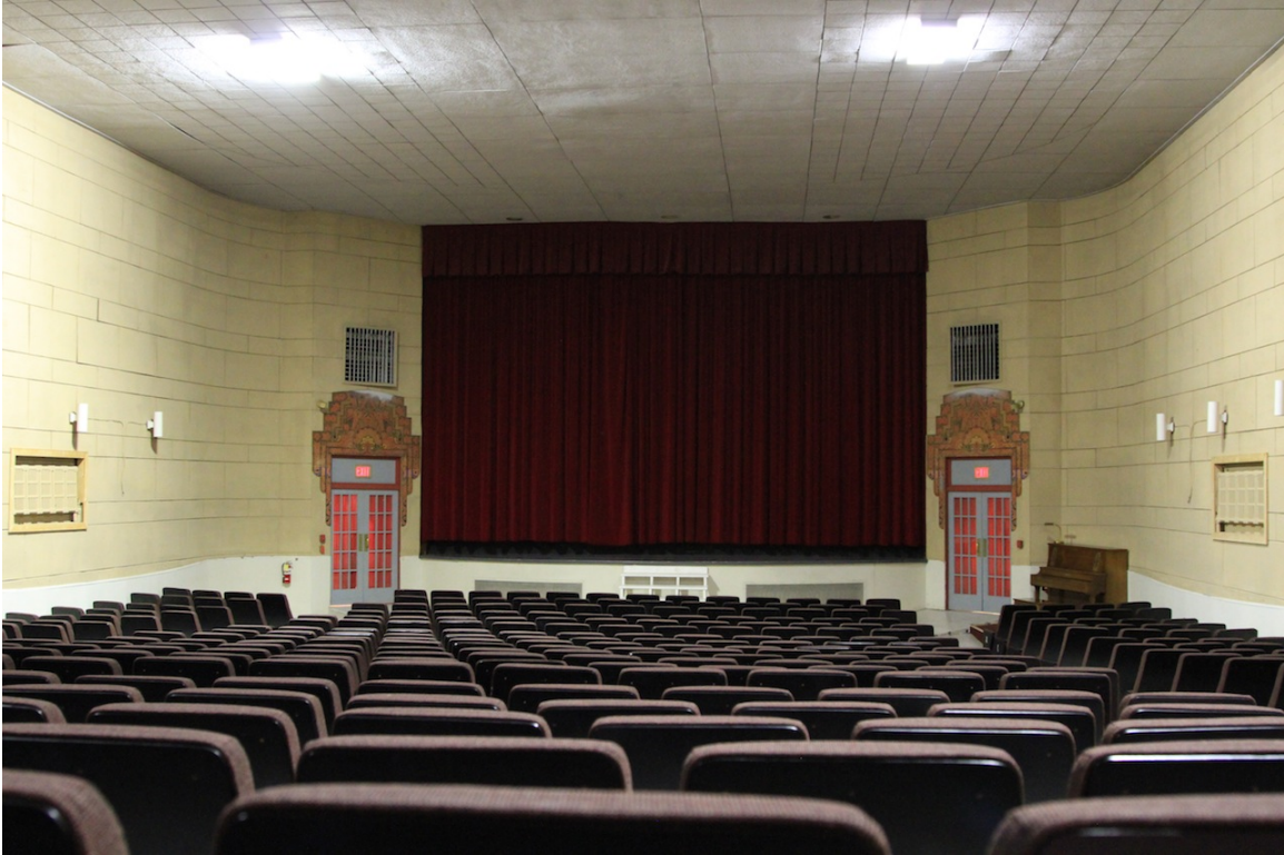
Theatre auditorium with twin double doors flanking a central stage from 1941 renovation. Note Donnacona acoustic panels on sidewalls (Donald Luxton & Associates, 2014).
