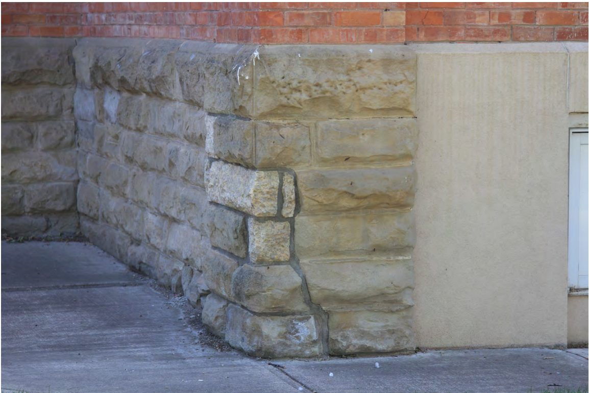
Area of sandstone and mortar repair and sandstone replacement at northeast corner of building. Note efflorescence where sandstone meets concrete pad, June 2015 (DLA)
