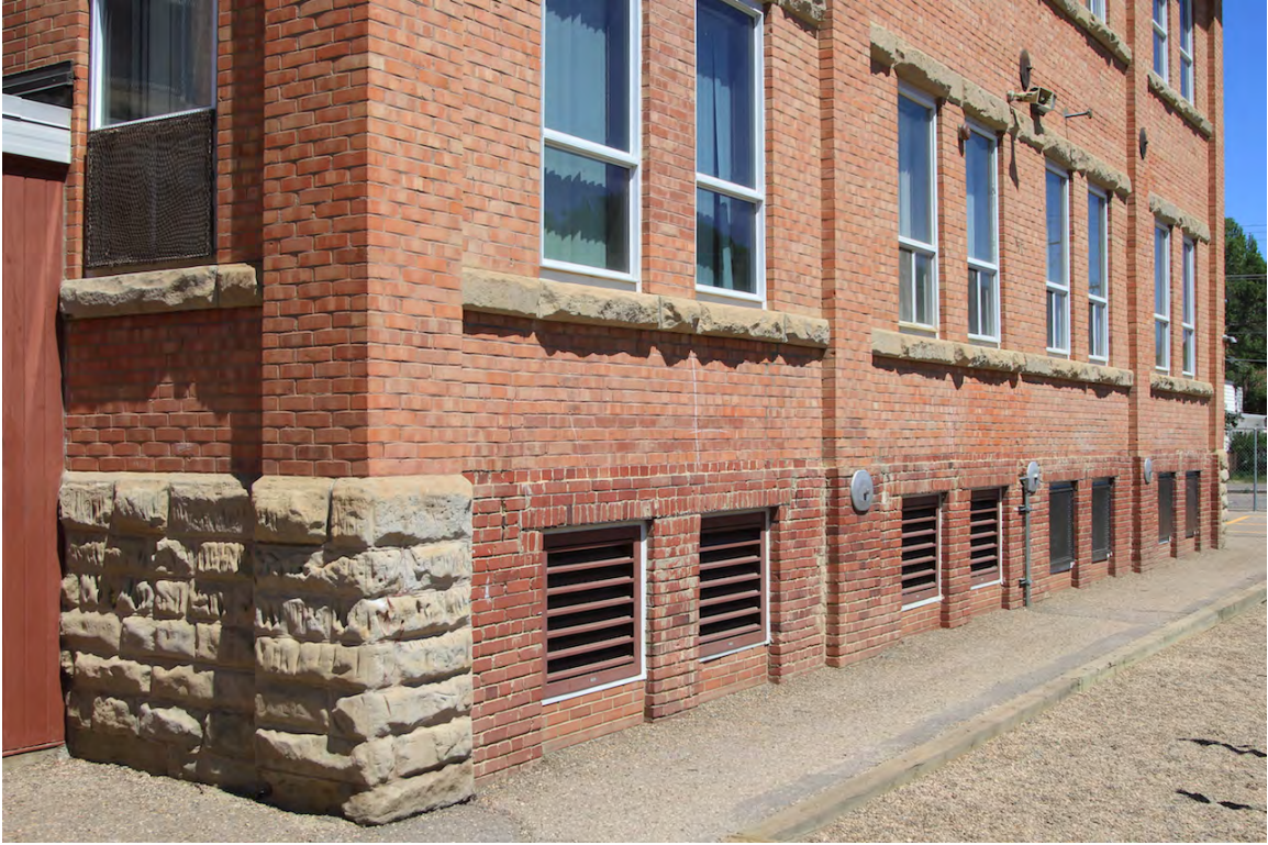
South façade showing sandstone replaced by brick, June 2015 (DLA)
