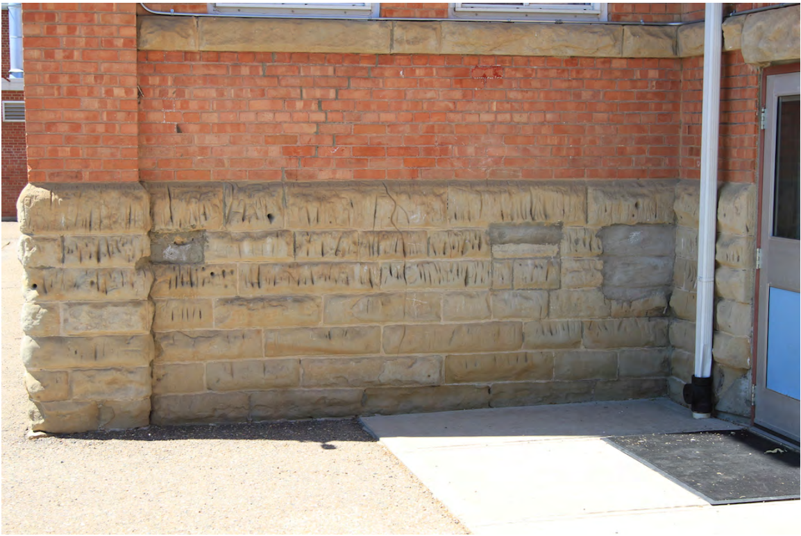
Southeast corner of school showing anthropomorphic damage and unsympathetic repairs to sandstone, June 2015 (DLA)
