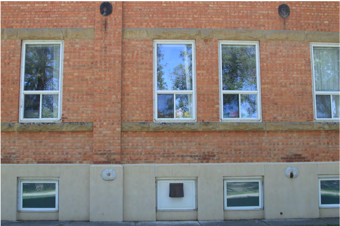
Front façade – full replacement of sandstone with concrete (parged), June 2015 (DLA)
