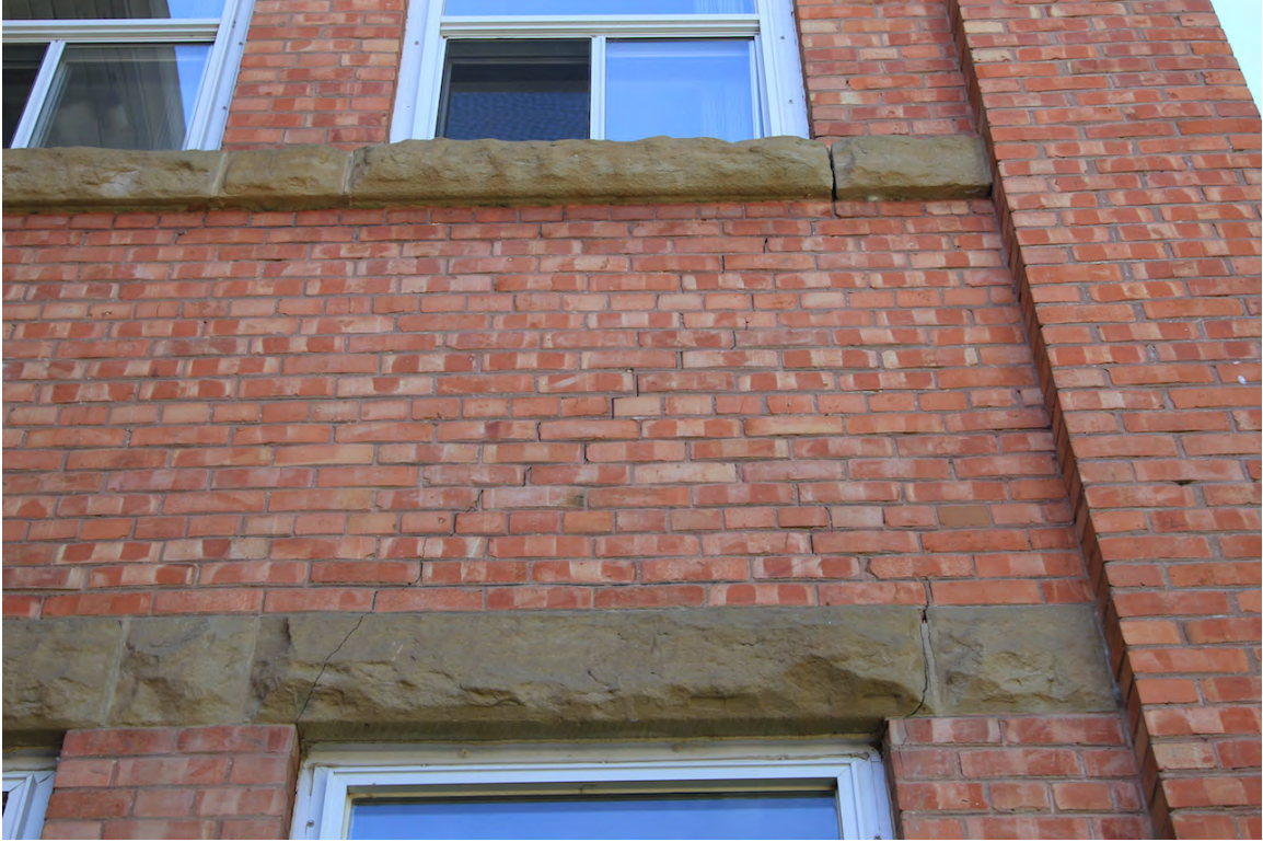
Cracking of sandstone from new window installation, June 2015 (DLA)
