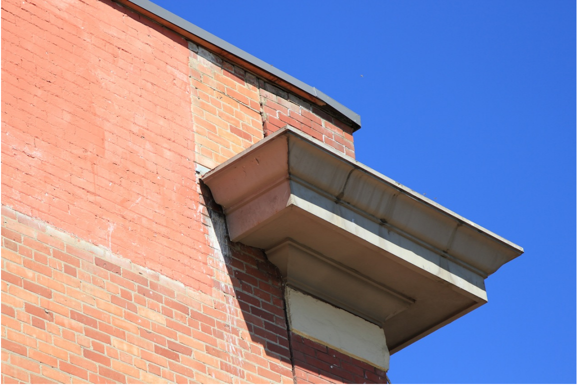
Hull Block – Pressed tin cornice and street façade and rear façade brick, 2014 (DLA).
