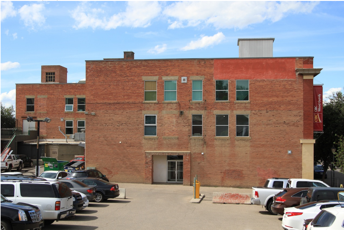
Hull Block – south façade showing original window fenestration, later added ground floor entry and bricked in window, 2014 (DLA).
