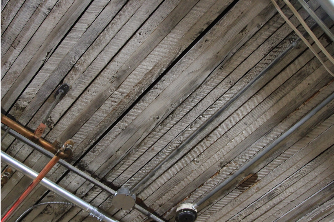
Hull Block – Underside of first floor laminated timber floor exposed in basement level, 2014 (DLA).
