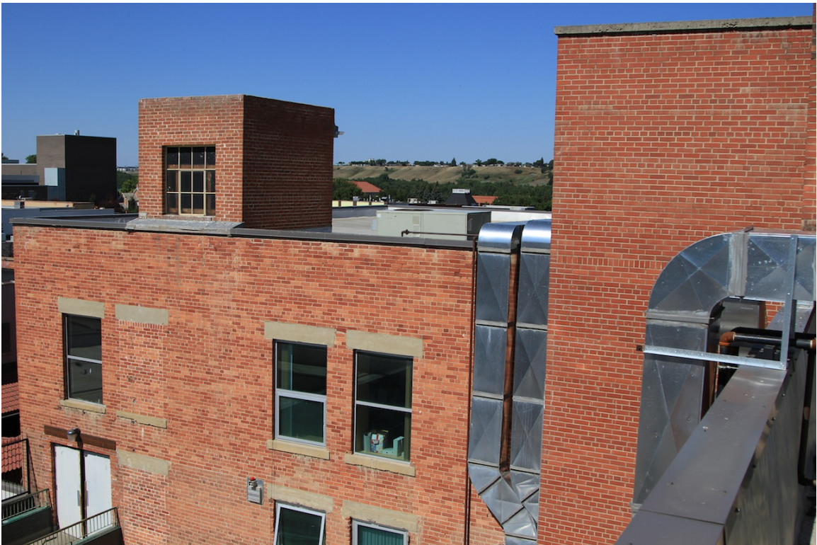
Hull Block – Later added brick elevator machine room on roof, 2014 (DLA).
