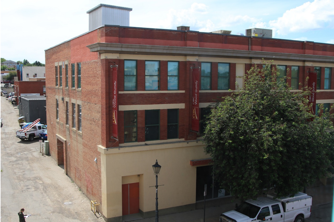
Hull Block – Structural bays separate by brick pilasters with triple assembly windows on second and third floors, 2014 (DLA).
