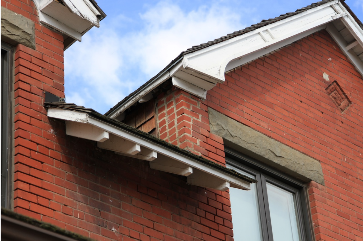
Mortar loss and past unsympathetic repointing on west elevation, June 2014 (Donald Luxton & Associates)
