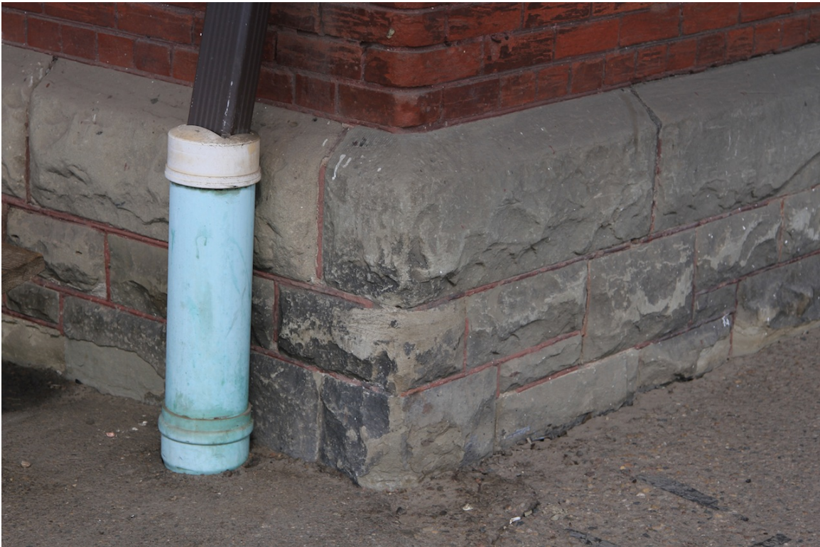
Stone water table with red mortar, June 2014 (Donald Luxton & Associates)
