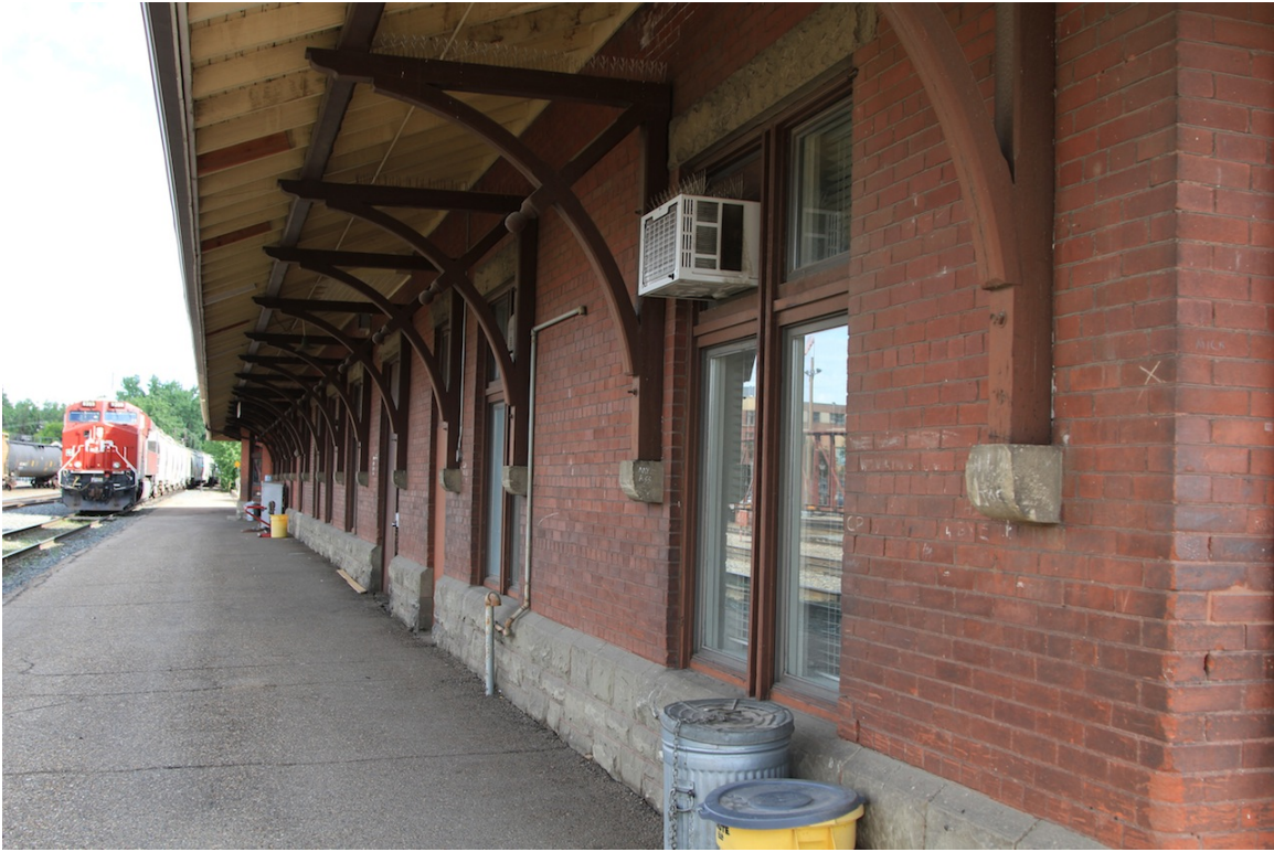
West side of station (by tracks) showing open soffits and brackets, June 2014 (Donald Luxton & Associates)
