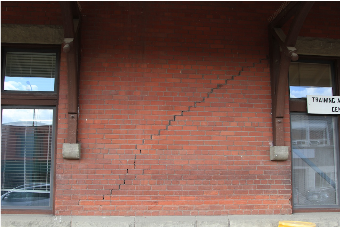
Cracking in mortar, west elevation of original building, June 2014 (Donald Luxton & Associates)
