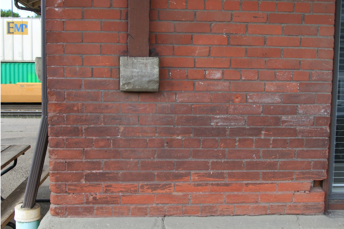
Mechanical wear on bricks from original portion of railway station (northwest side, facing tracks), June 2014 (Donald Luxton & Associates)
