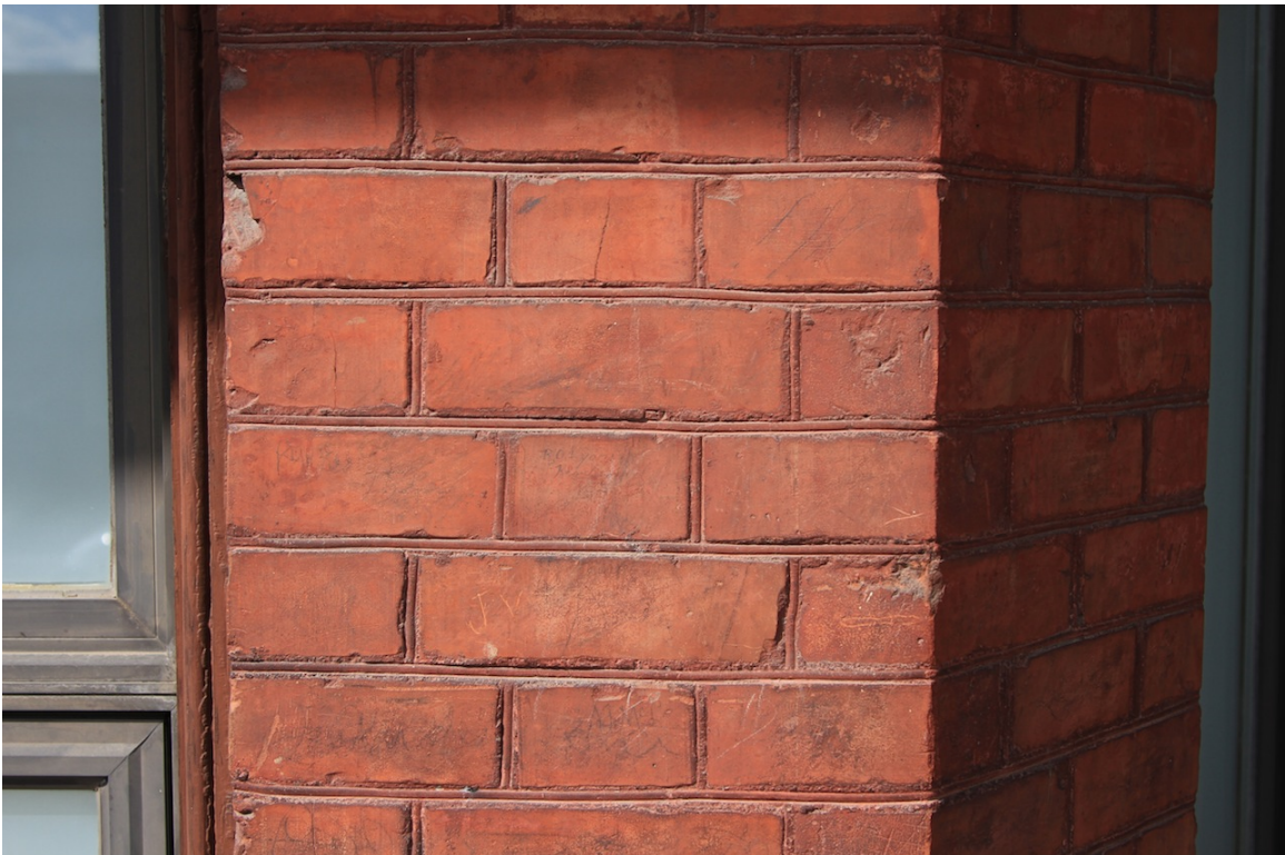
Close-up of bricks with tooled mortar – original building (northeast corner), June 2014 (Donald Luxton & Associates)
