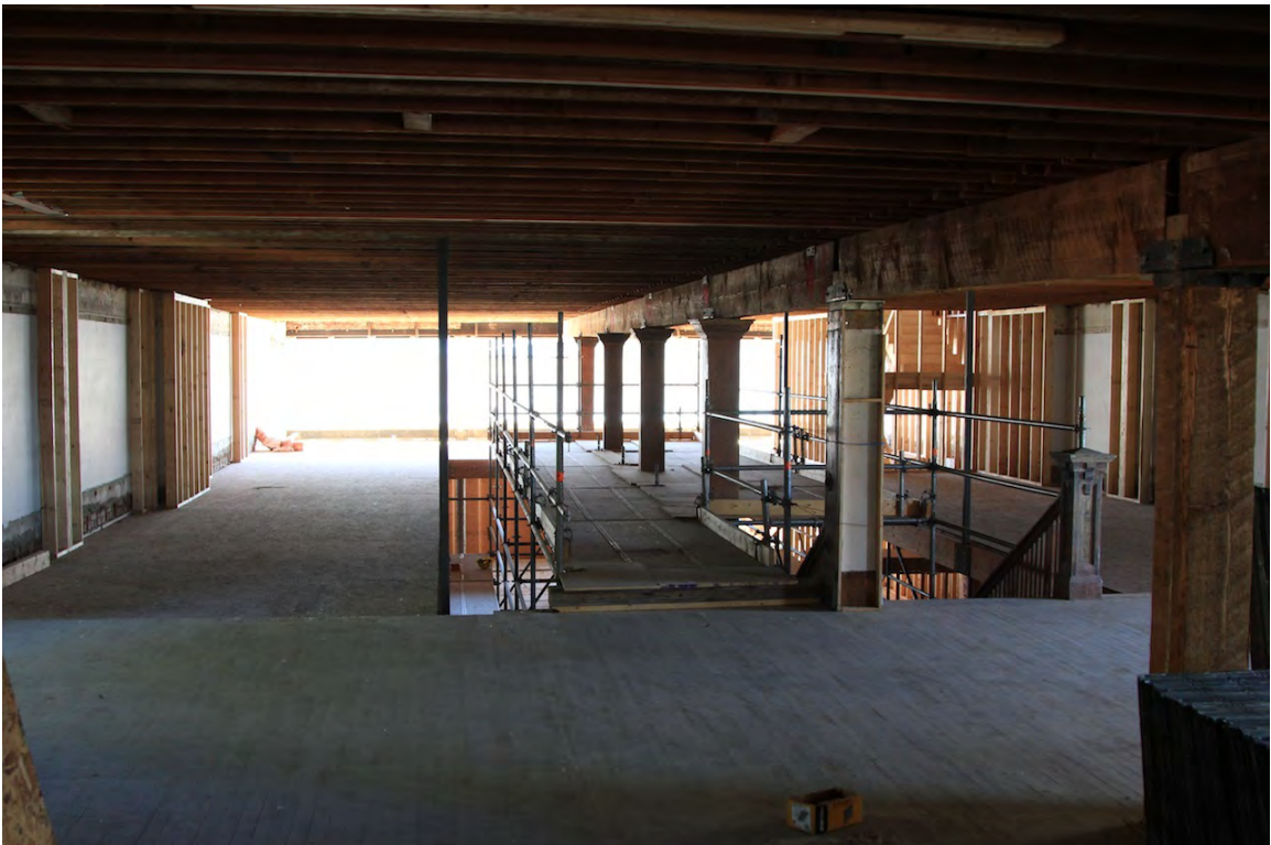
Mezzanine level with original wooden floor and wooden columns, 2014 (DLA)
