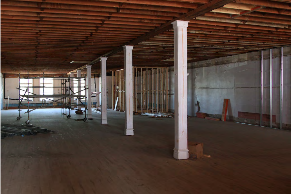
Second floor with original wooden floor and columns, 2014 (DLA)
