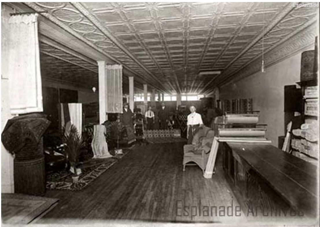
Interior of Beveridge Block showing second floor circa 1910s (Esplanade Archives)
