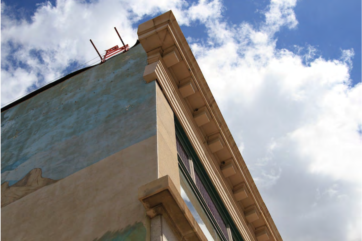
Corbelled architrave and substantial pressed tin cornice with modillions, 2014 (DLA)
