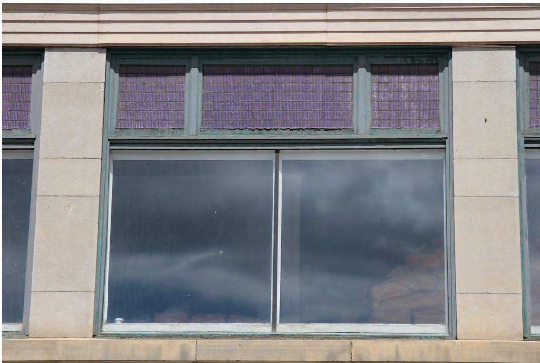
Second storey fixed tripartite wooden-sash window with amethyst glass transom, 2014 (DLA)
