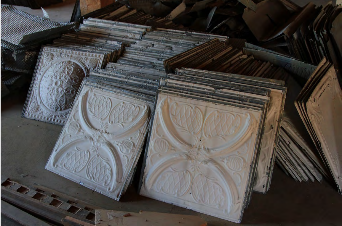
Removed pressed tin ceiling tiles, 2014 (DLA)
