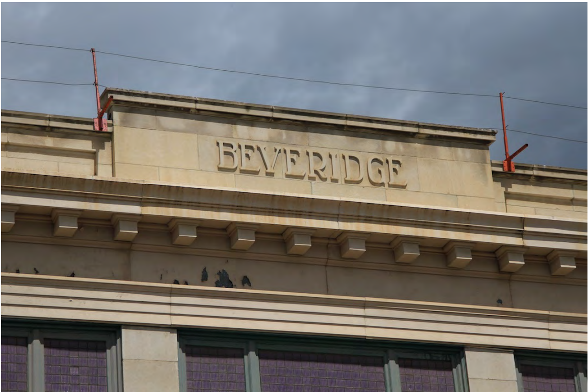
Stepped capped parapet with central signband, 2014 (DLA)
