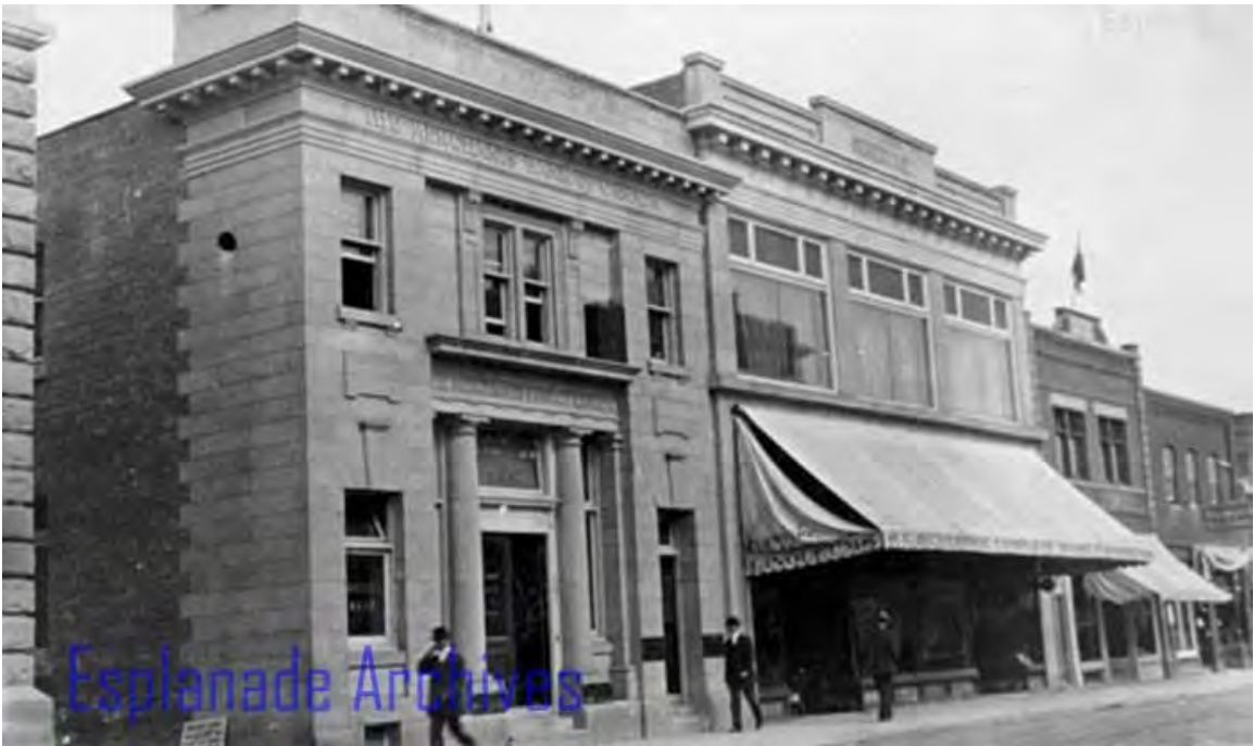
Beveridge Block (centre with large awning), 1913 (Esplanade Archives)
