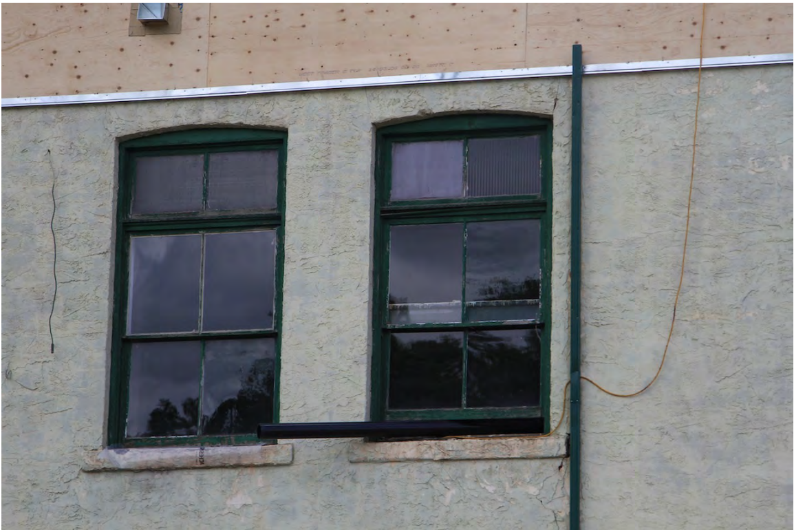
Segmental arch 2-over-2 single-hung wooden-sash window with reed glass transom, 2014 (DLA)
