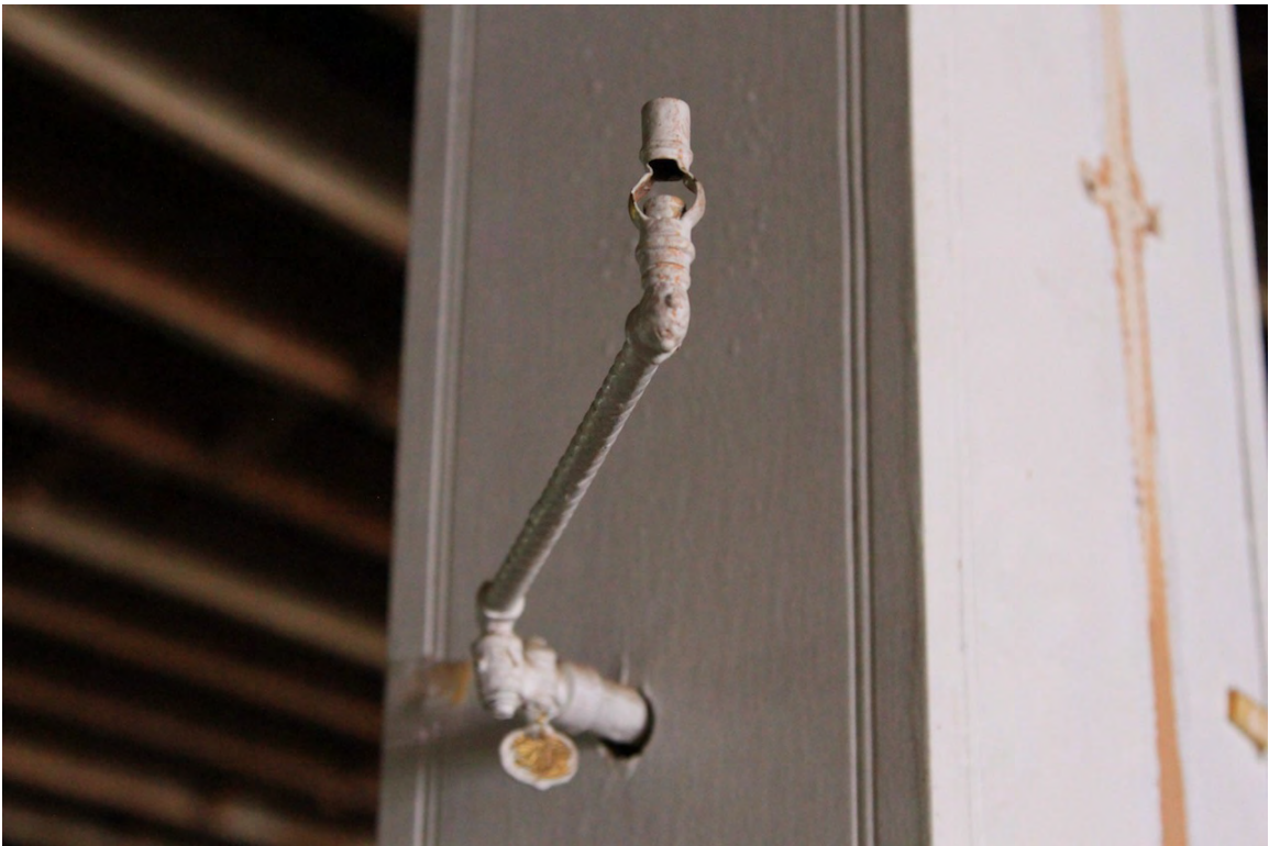
Gas light fixture on wooden column, 2014 (DLA)
