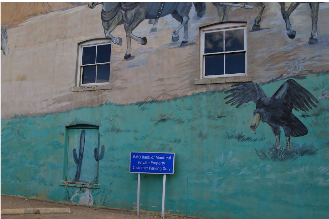
Segmented arch single assembly 2-over-2 single-hung wooden windows on west façade, 2014 (DLA)
