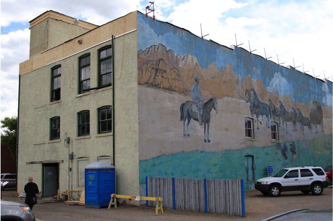
North and west façades of Beveridge Block, 2014 (DLA)
