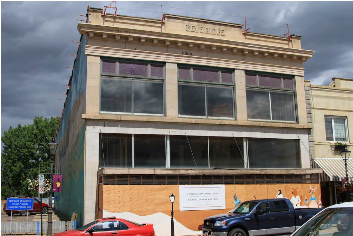
Street façade of Beveridge Block with full-width transom on first floor and three structural bays on second floor, 2014 (DLA)
