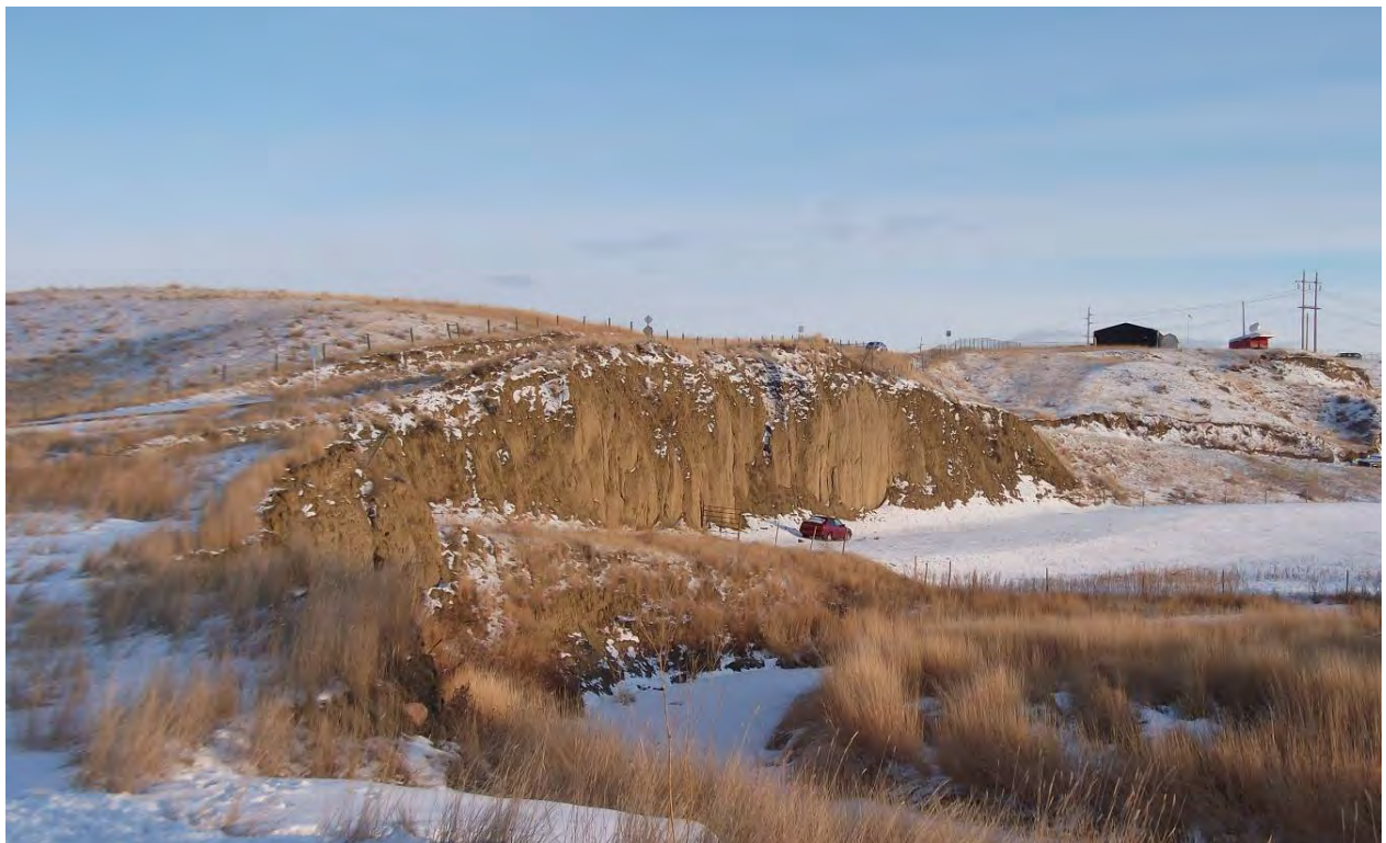
Photograph 18: Looking east at the east side of Route 6 alignment. Note the vertical eroded face adjacent to the existing roadway.
